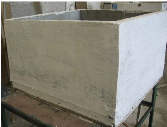
Figure 3. Healthy Ferrocement Tank.
