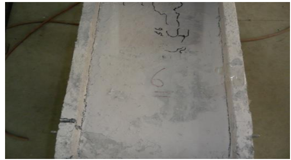
Crack pattern of S6
