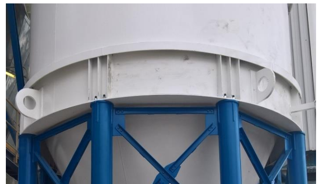
Fig. 2. Stiffening elements above discrete supports of the shell.
