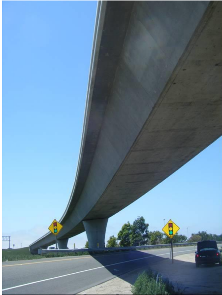
Fig. 2. A close look of the Fairview Road On-Ramp Overcrossing (FRO) Bridge.
