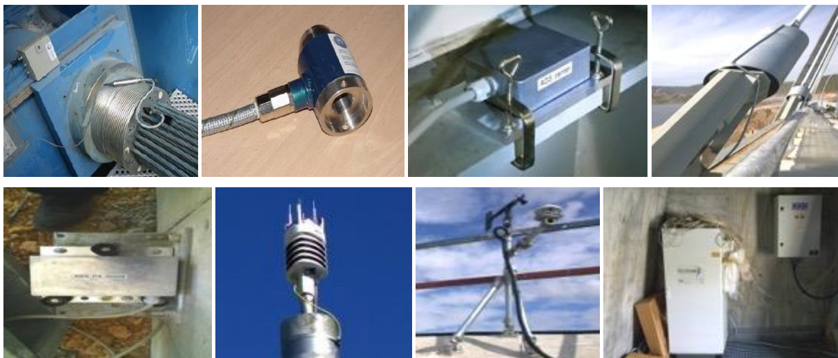
Fig. 3. Some views from sensors located in Nissibi Bridge (NBR, 2015).
