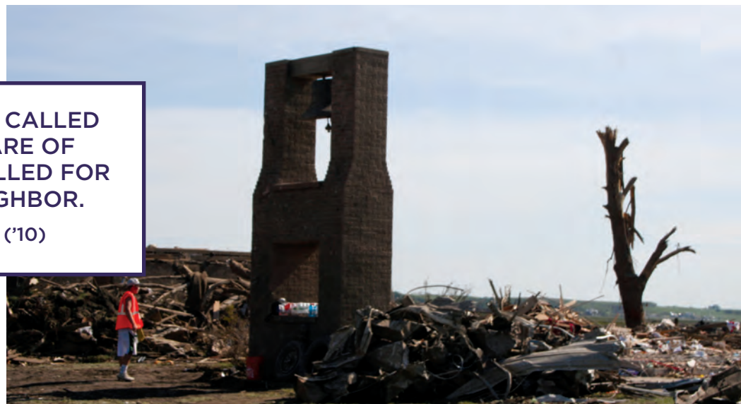
A tornado leveled St. John's Lutheran Church in Pilger, Neb., in June 2014. The only structure left standing was the church's bell tower. Photo: Courtesy St. John's Lutheran Church
