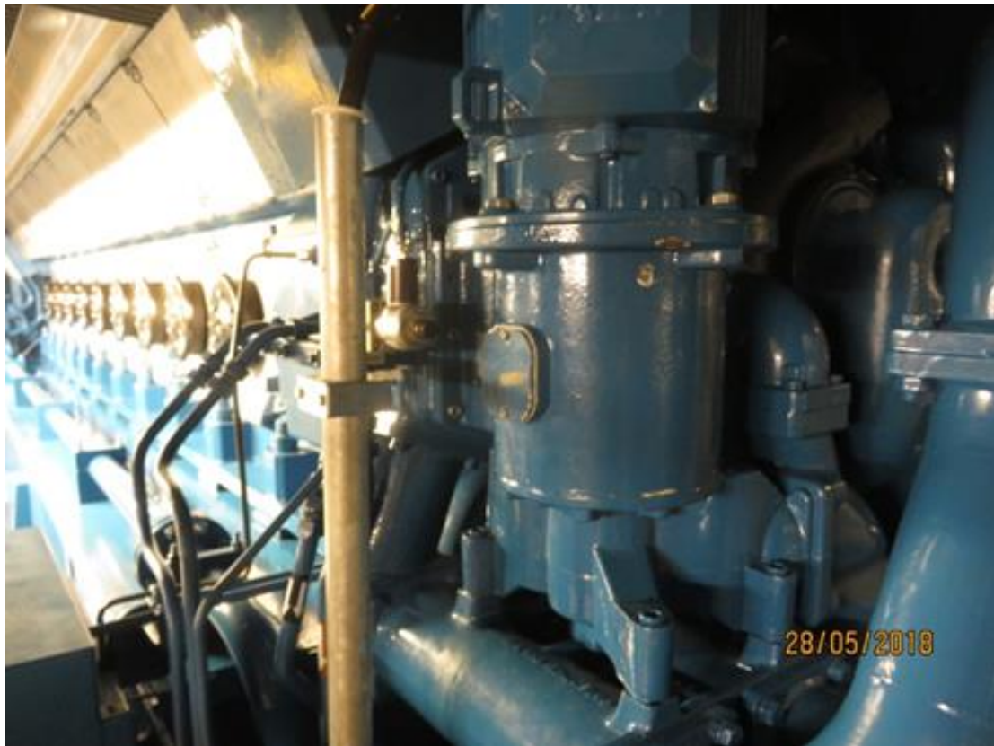
Figure 2.1 Pre-lubricating gear pump Kracht
