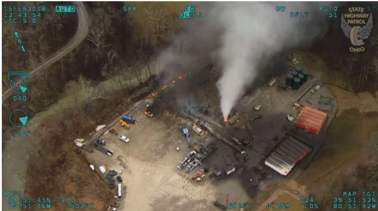
Figure 16. XTO Energy Schnegg well pad blowout that occurred on February 15, 2018 (Ohio State Highway Patrol, 2018).
