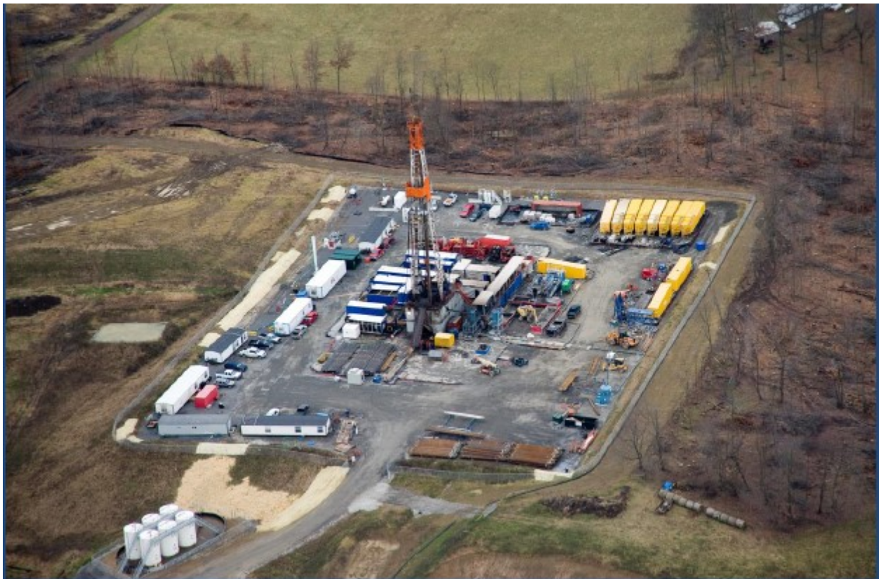
Figure 5. Well pad set up in Ohio (Ohio EPA, 2017)
