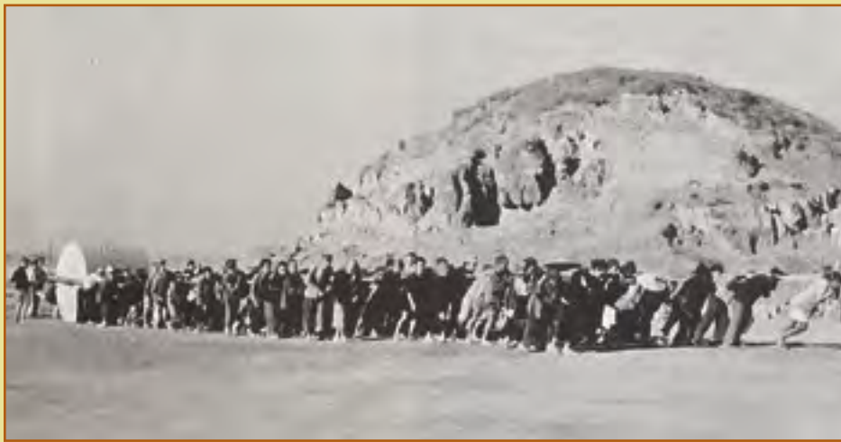
Workers constructing an airfield in China
