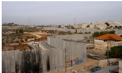
Figure 2.1c. Walled in camp with tower at fore; same camp as below. (copyright free) http://travel.mongabay.com/kenya/images/kenya_elf_0032.html
