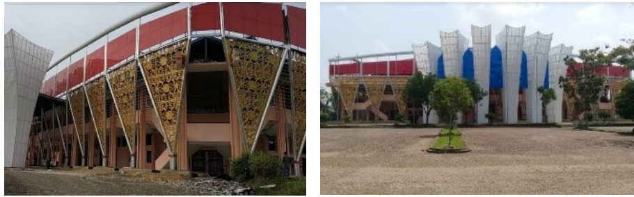
Figure 3.8. Kota Baru Jambi Sport Building (Hamidah, 2019)
