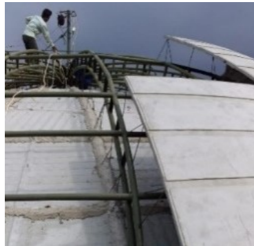
Figure 3.20. GRC Framework and Panel (authors, 2019)
