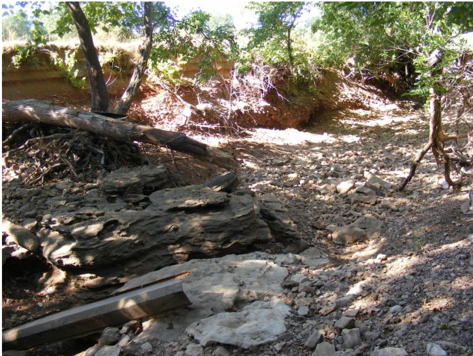
Photo 8. Bedrock Knickpoint #2 (2,900 ft) looking at the left bank erosion near the second knickpoint on the north property.
