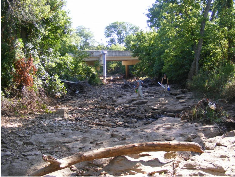
Photo 1. Bridge Reach (3,850 ft) looking upstream at USGS gage at FR 156.
