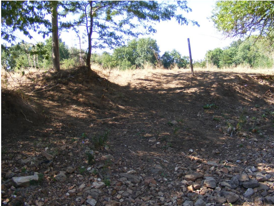
Photo 10. Cattle damaged banks (2,600 ft).
