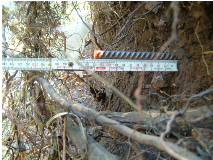
Photo 4. Measuring bank erosion at a pin
