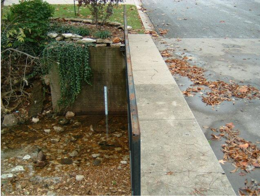
Photo 3. Site 3 downstream of bridge at Camino
