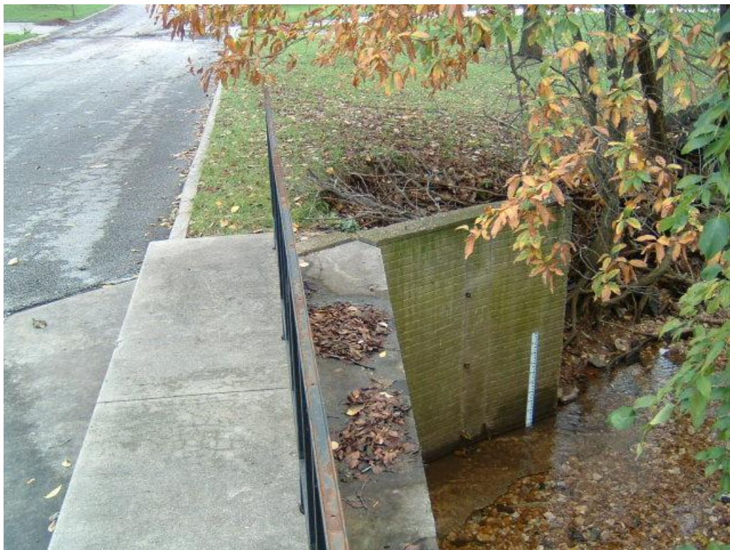
Photo 2. Site 2 downstream of bridge at Holland
