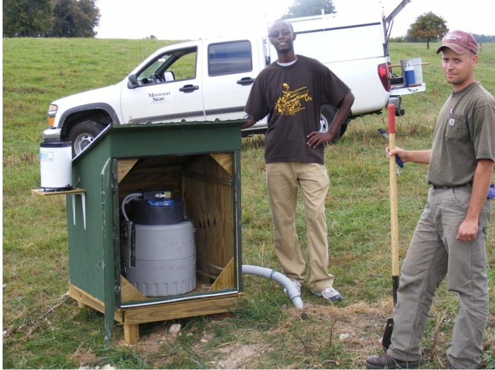
Photo 5. Auto-sampler and Rain Gage Installation (October 2008)
