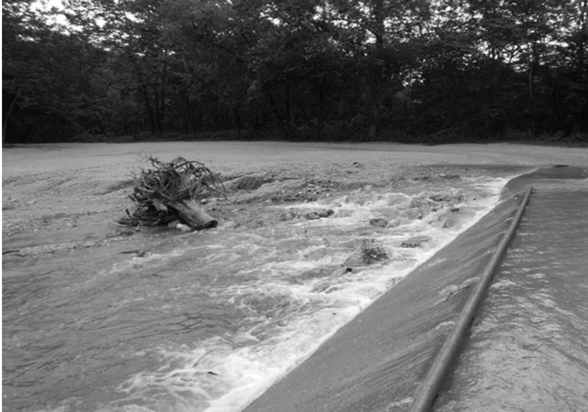
Figure 4. Image of the lateral overflow formed along the edge of the main channel crossing during moderate flows. The discharge at Akers Ferry was approximately 28 \text{ m}^3/\text{s} during this photo. Photo taken 17 August 2017.
