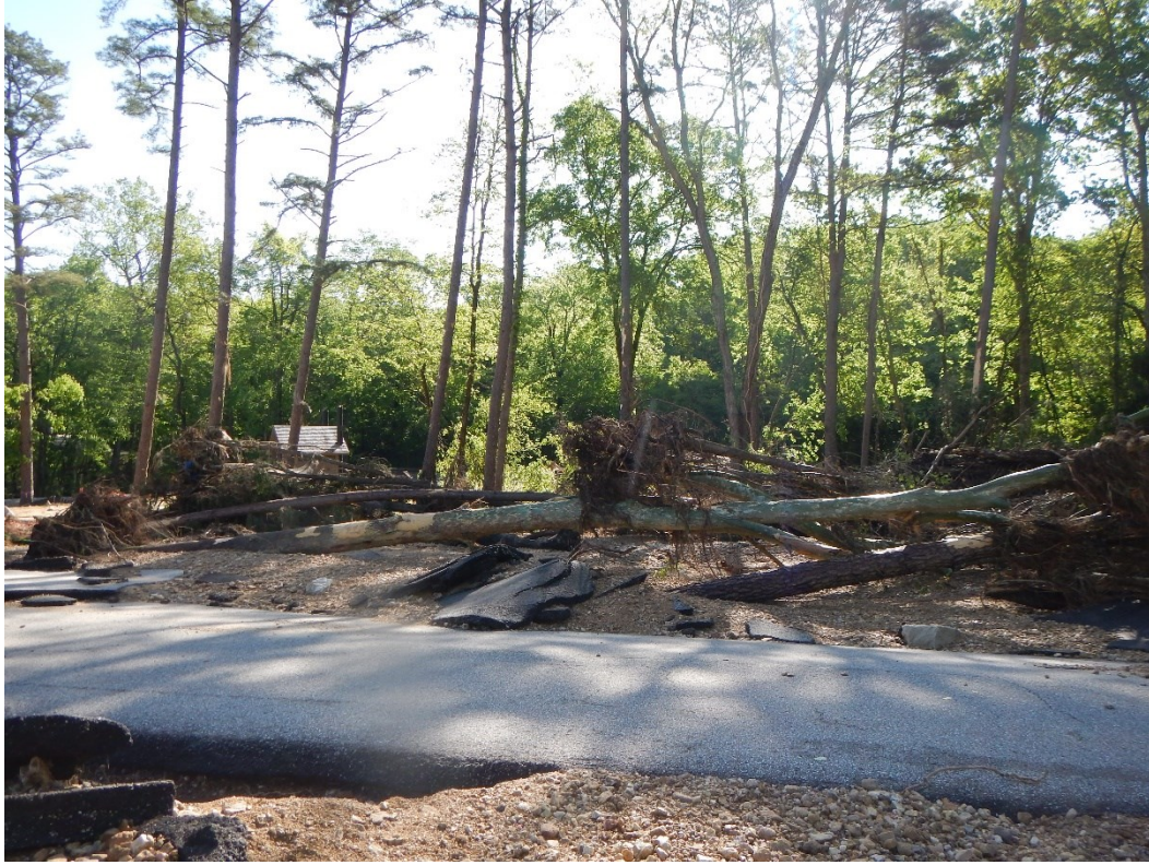
Figure 55. Imbricated asphalt pieces and toppled riparian trees caused by the April Flood.
