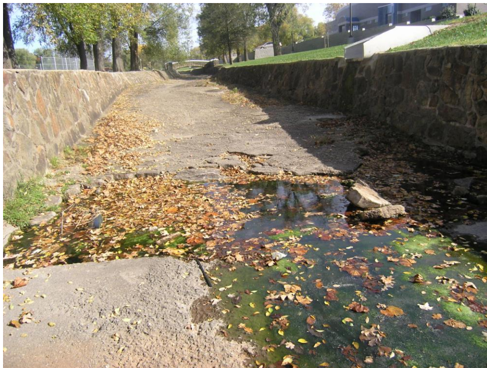
Site NB1: Upstream view showing dry channel and karst seep
