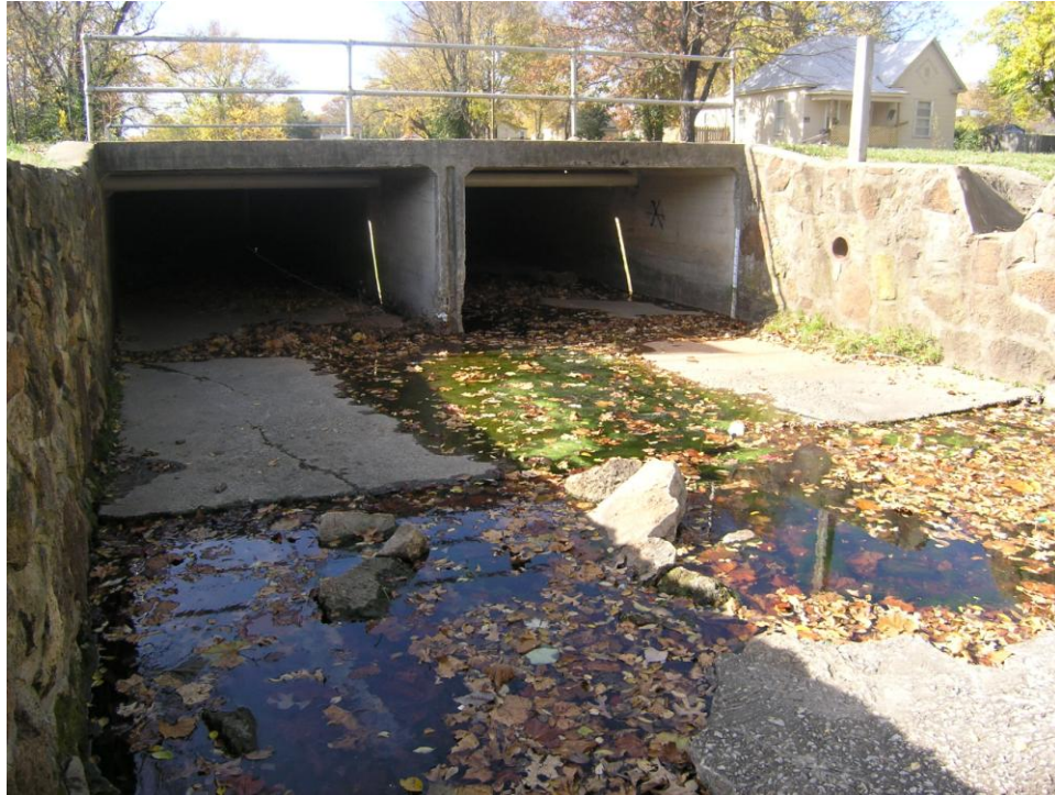
Site NB1 (North Branch Jordan at Fremont Ave): Downstream view showing gage location, dry channel and karst seep
