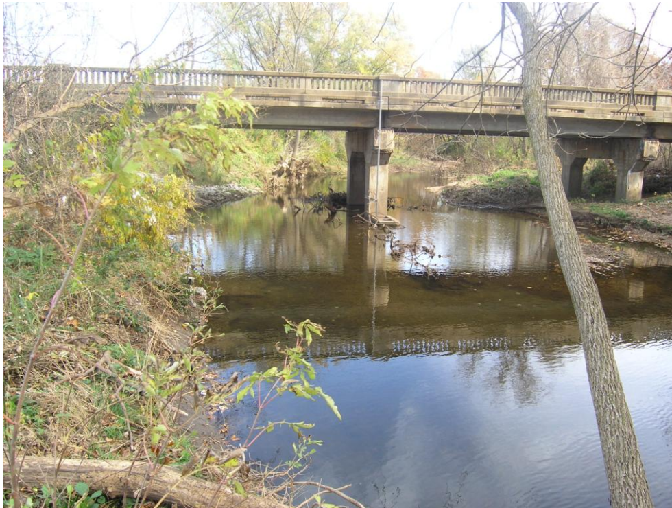
Site WC1 (Wilson Creek at Scenic Avenue): Upstream view showing baseflow. USGS gage is obscured by foliage at right of photo, gage sensor pipe on central bridge pier
