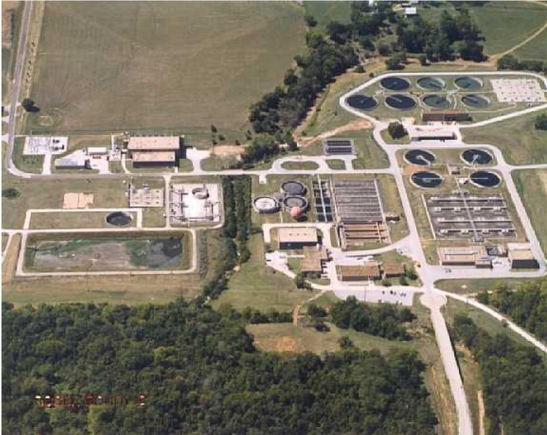
Figure 14. Springfield's Southwest Wastewater Treatment Plant (used with permission).
