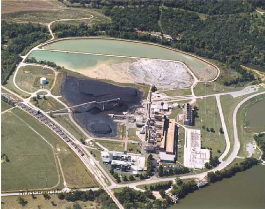
Figure 15. Springfield's Southwest Power Station (used with permission).
