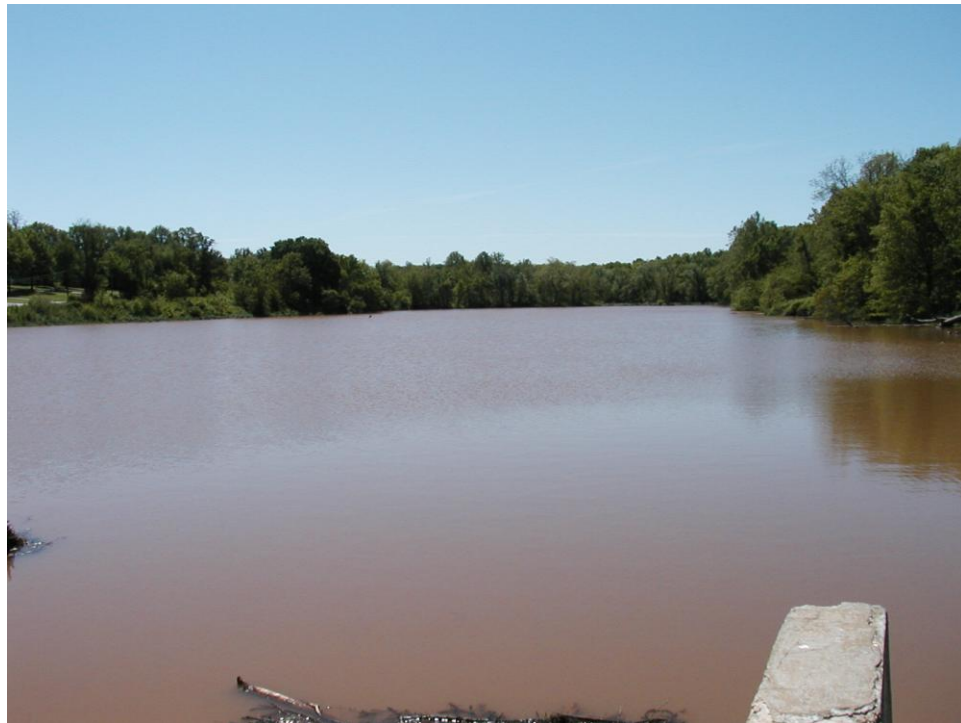
Figure 3.2 Valley Mill Reservoir with Water Level at Full Pool
