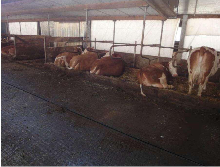
Figure 9: Yard in commercial dairy farm 3 with deep bedded free stalls and grooved concrete flooring.
