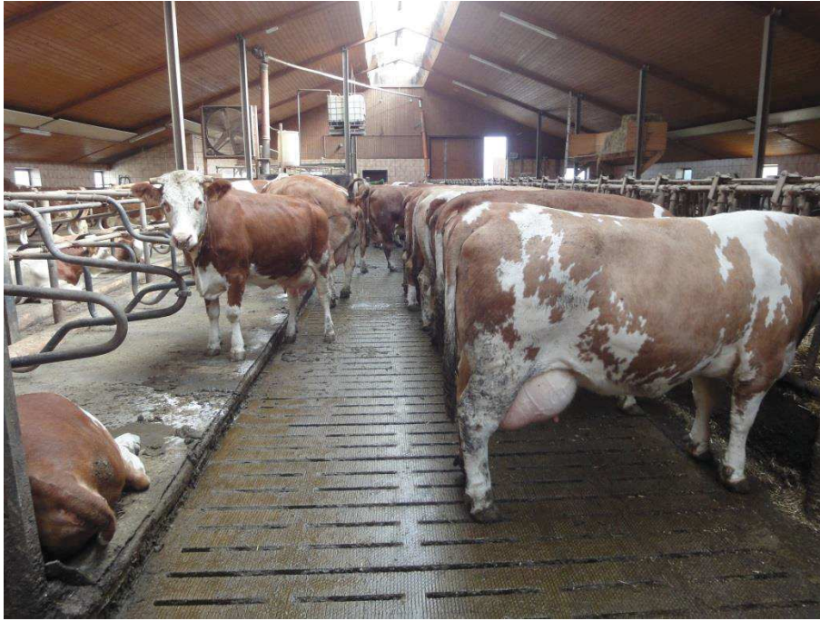
Figure 6: Slatted concrete flooring and concrete free stalls with rubber mattresses on commercial dairy farm 2.
