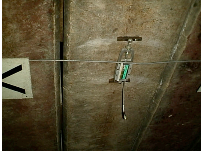
Figure 3 – Demountable strain gauge attached to bridge soffit.
