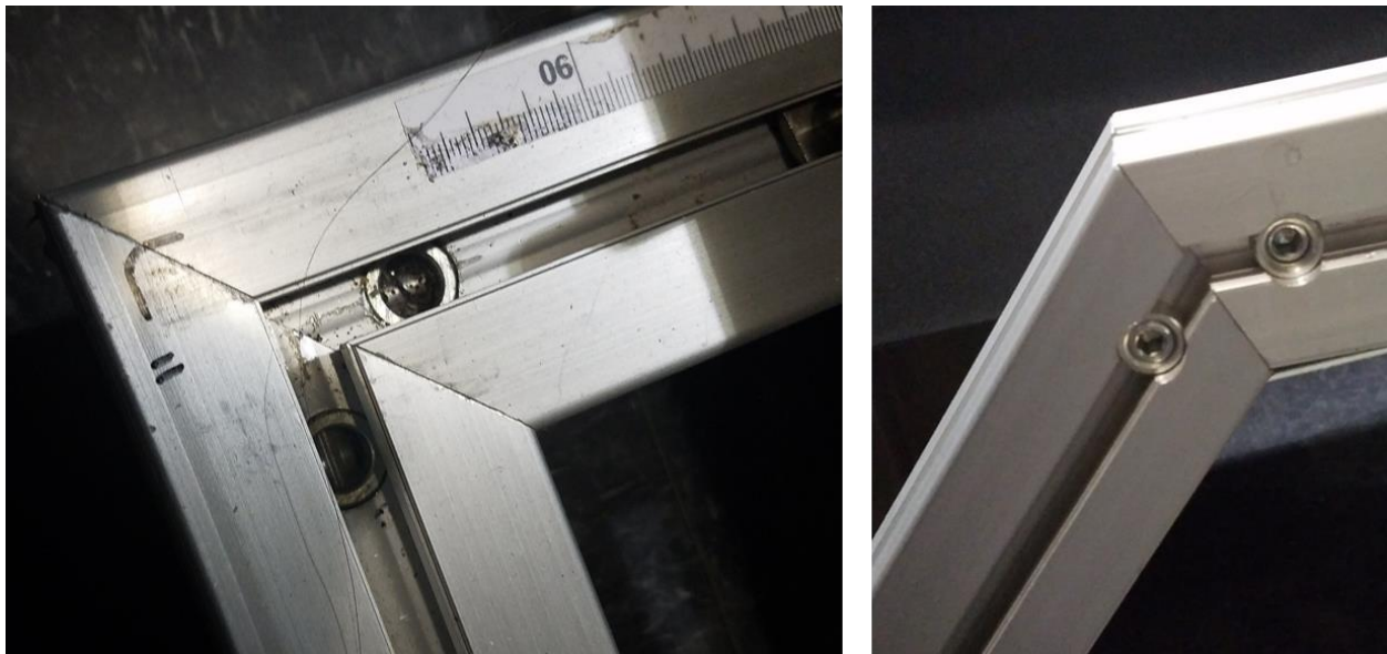
Figure 94: Examples of joints on the frame with embedded pins and locking bolts.
