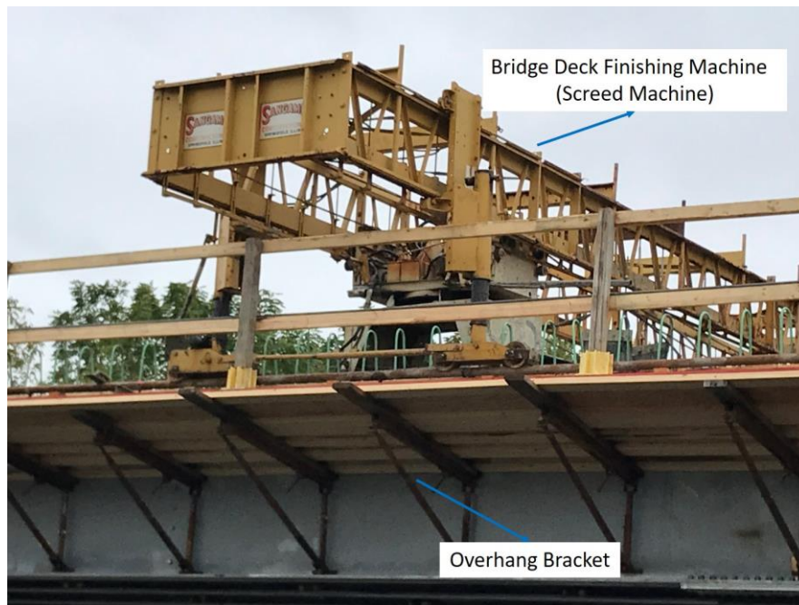
Figure 1. Construction of deck overhang.
