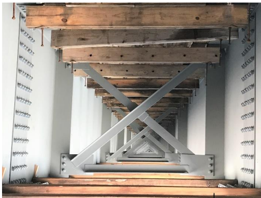
(a) Cross-frame with full-depth connecting plate
