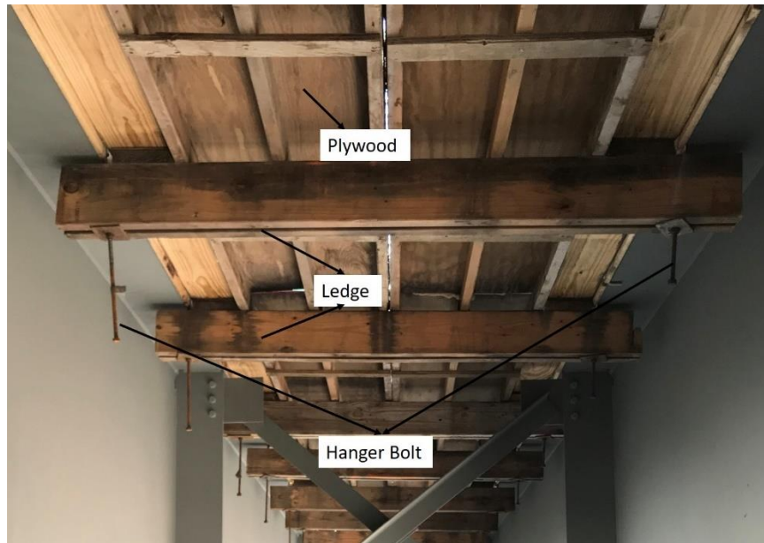
Figure 4. Interior formwork.
