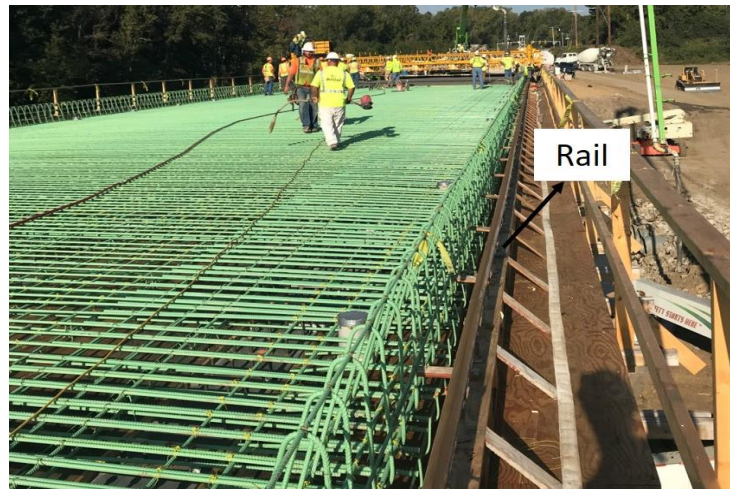
Figure 7. Screed-machine rail located outside the exterior girder on the overhang.
