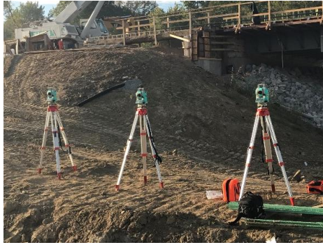
(a) Total station
