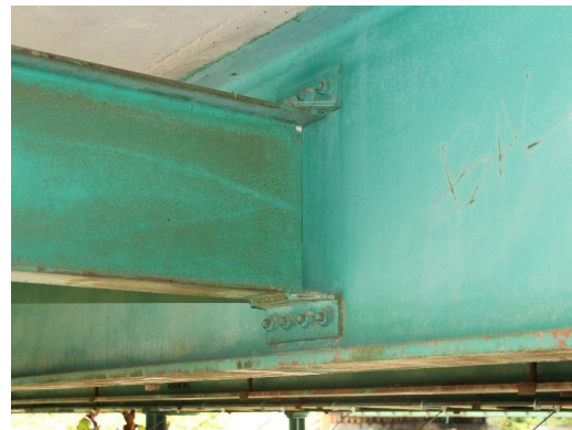
(b) Diaphragm with angle steel connection
