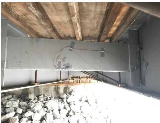
(c) Diaphragm with partial-depth connecting plate
