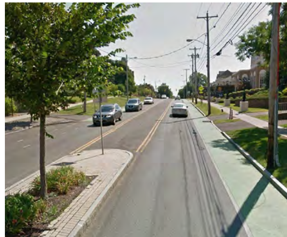
Figure 23. Genesee Street in Syracuse, NY. This is a reconstructed commercial street in a traditional setting. A dedicated bike lane along with fewer and thinner drive lanes creates a safer environment for cyclists. The sidewalks are also pulled back from the street creating a more comfortable experience for pedestrians (Image credit: Google Maps).
