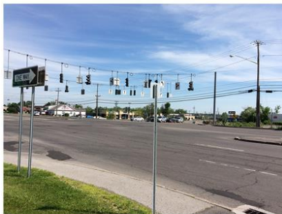
7-8 lane intersection at Bridge St..JPG
