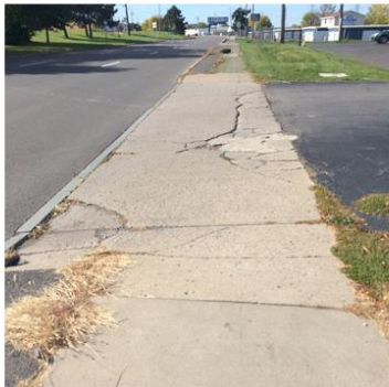
Crumbling sidewalk.jpeg
