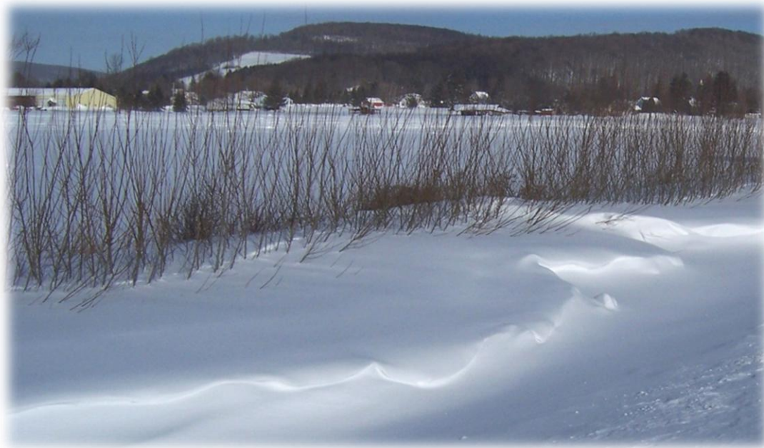
Snowdrift formed downwind of a three year old shrub-willow fence on Interstate 81 in Preble, NY
