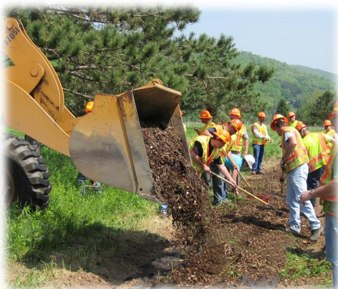
Figure 5 (left) – Applying wood mulch to a planted shrub-willow snow fence Figure 6 (right) – Planting cuttings directly through mulch and landscape fabric underneath Photos by SUNY ESF
