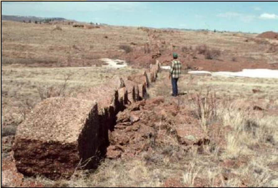
Rock snow fences protecting a railroad cut in SEW Wyoming were probably built in 1868 (Tabler 2003)
