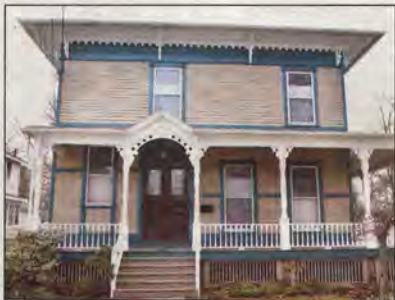
306 Main Street is a prime example of a well-preserved 1886 home of Italianate style with some very special features. It has two curved bay windows strategically placed to capture sunrises and sunsets. The most striking feature of the interior of the house is the large array of hand-painted, ornamental and pictorial murals by David Bruce, a well-known artist who died in 1905. Provided photo.
