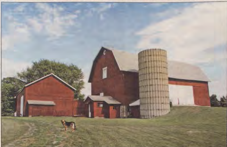
In the Dilger barn complex, the barn at the left is estimated to date back to the mid-1800s and the large barn to circa 1900. With a crumbling foundation wall under the facing white door, Hank Dilger and a crew went into action last spring. Old rocks were hauled out, a 35-foot steel I-beam was inserted, a foundation was dug, a concrete block foundation was erected, and a new concrete apron poured in front of the white door. In the foreground is their beloved dog, "KD" (pronounced Kadey). Photograph by Dianne Hickerson.
