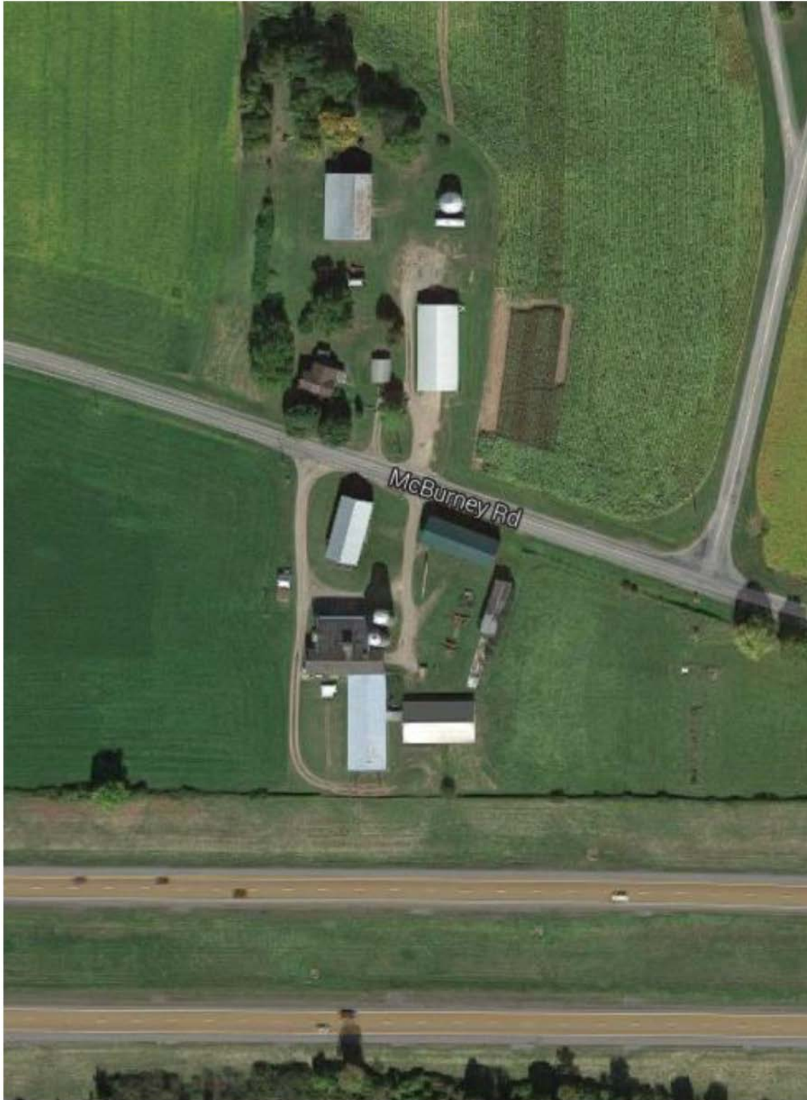
Figure 3: View of Franklin Farm from the air. Image via Google Maps. Well house visible as small white roof; bottom-left most building.
