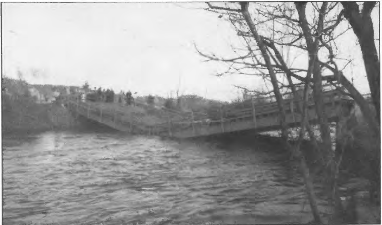
Figure 6.--Collapsed Osceola Bridge during flood on the Salmon River in Osceola, December 29, 1984. (Courtesy of Carroll E. Owens.)
