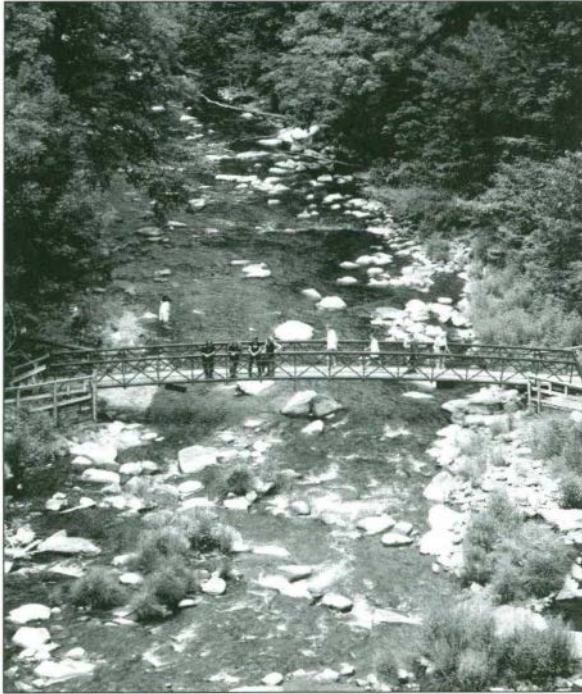
Bridge over Chittenango Creek (Photo: Saltman)
