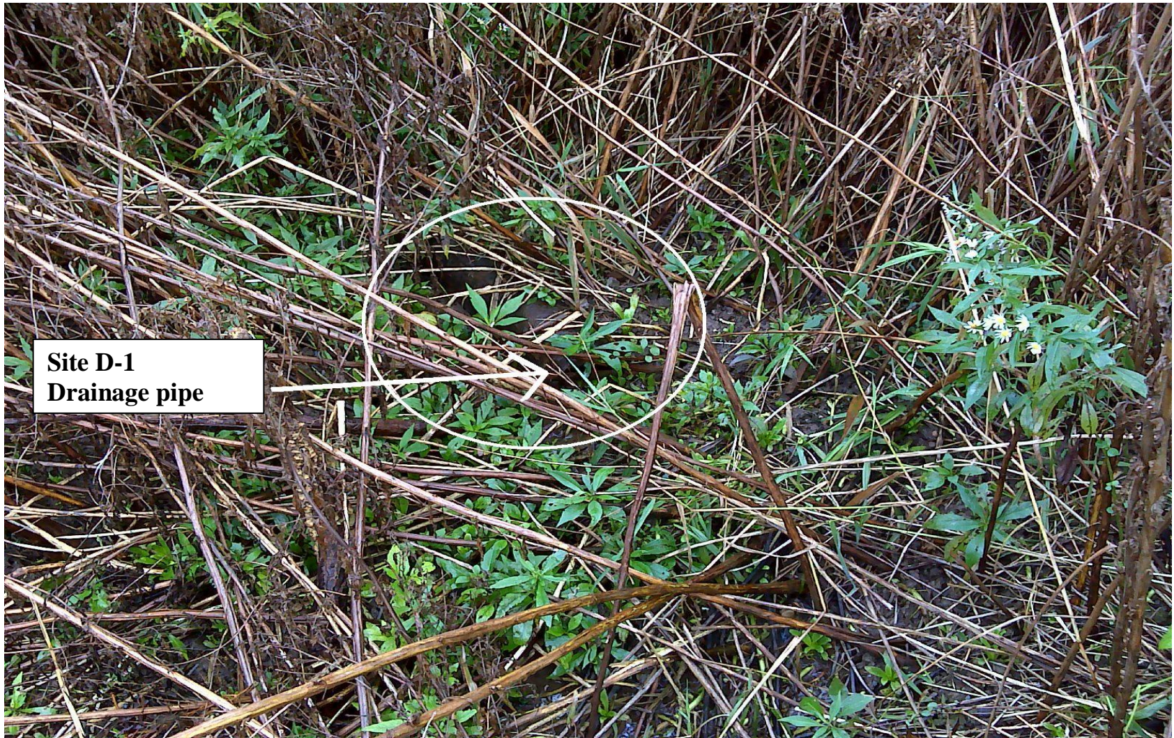
Figure 41. Picture of Site D-1 in the Wyoming Road subwatershed (Fig. 38), Drainage pipe feeding out from under a residence.
