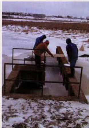
FISHWAY CONSTRUCTION AT OSHAWA SECOND MARSH, IN WINTER
