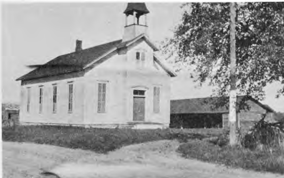
OLD METHODIST CHURCH - WEST SWEDEN
