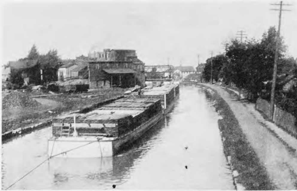
The Erie Canal was the connecting link with ports on the Great Lakes in the west and coastal cities in the east. This view looks west toward Main Street and shows the "Erie" before it was widened. Note the tow path along the north bank, also many buildings which have disappeared.
