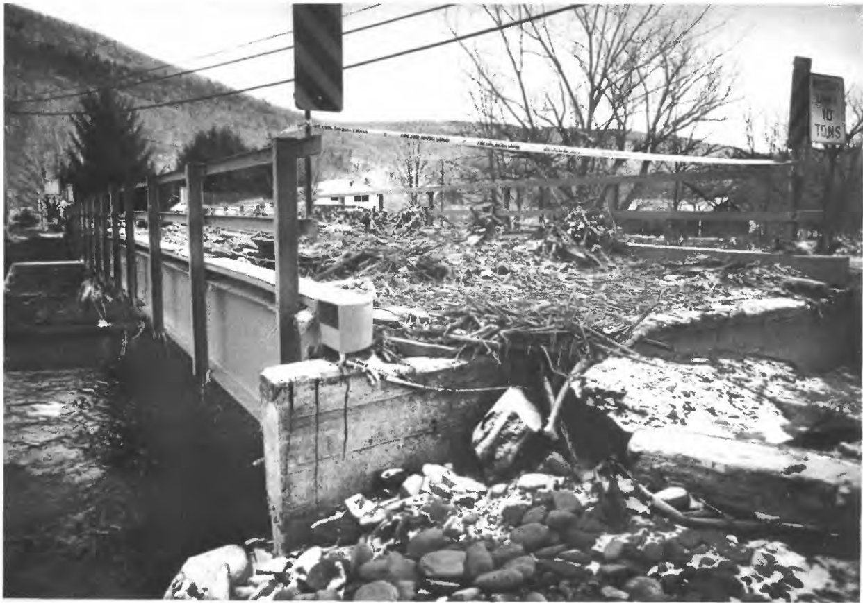
Figure 9B. Fair Street bridge over the East Branch Delaware River at Margaretville, N.Y. after the flood of January 19, 1996 (Photograph courtesy of the Oneonta Daily Star, January 30, 1996, p. 8.)
