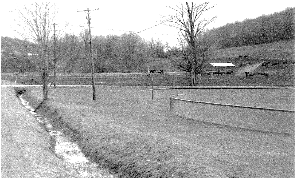
Figure 7. Ditch that runs into a culvert at site 16. Note extensive area of exposed soil in pasture of grazing horses.
