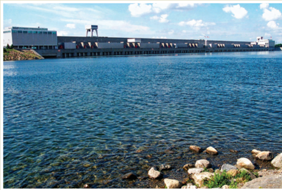
Moses Saunders Power Dam on the St. Lawrence River between Massena, New York, and Cornwall, Ontario.
