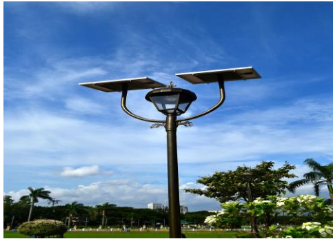
Fig4.2 Solar cells street lamp
