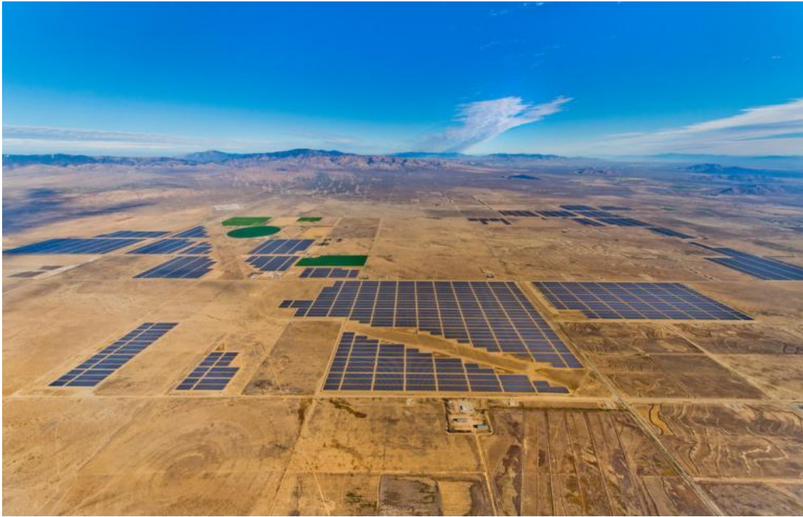
Fig 4.31 Overlook at the Solar Star
