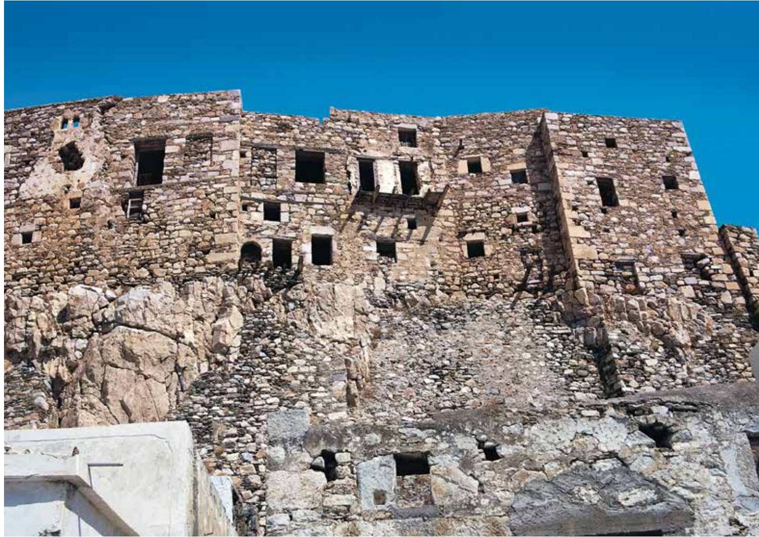
Astypalaia, Kastro, exterior walls. The absence of any traces of stucco or whitewash might serve to reinforce the argument that on earlier days the exterior walls of a Kastro were not whitewashed, allowing the mass of the edifice to merge visually with its immediate surrounding and escape the observation of pirates. In contrast to the practice of Sifnos Kastro, here the exterior walls and roofline do not reveal the specific location of individual interior dwelling units.
