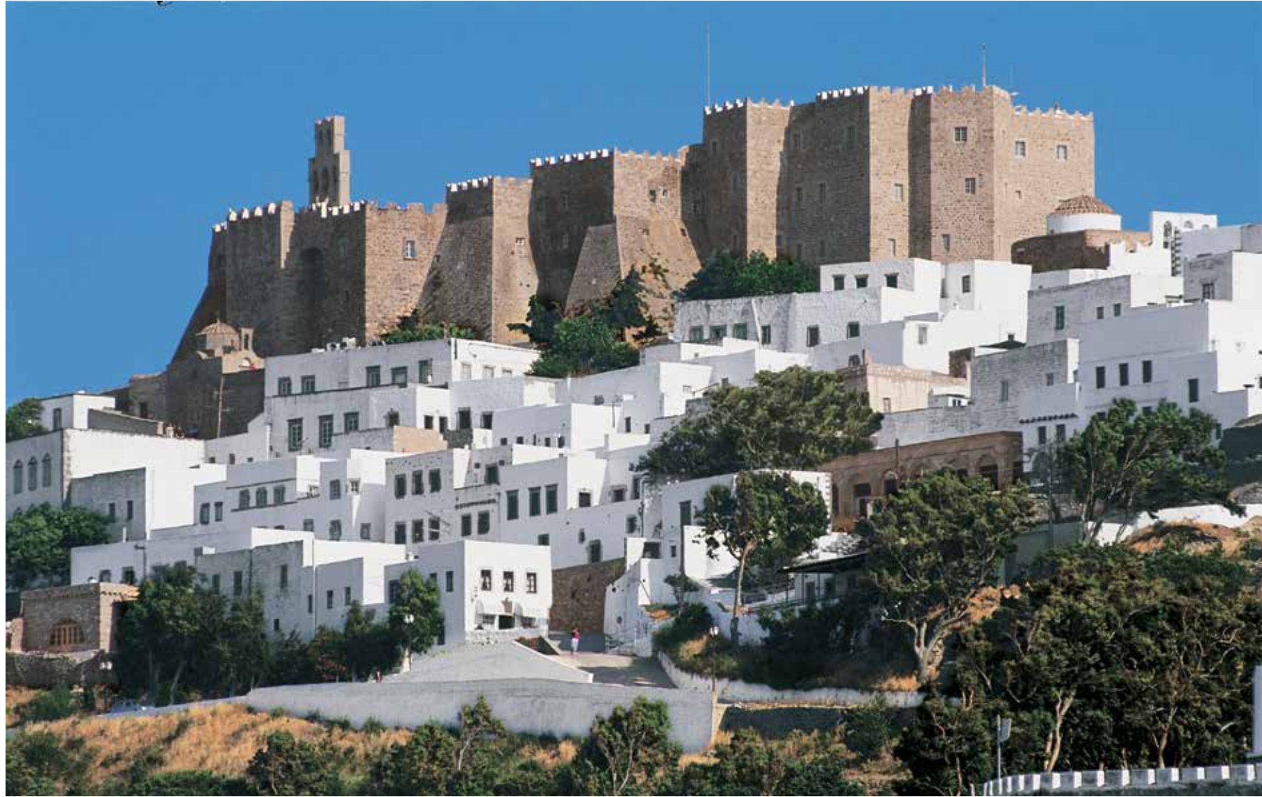
Patmos. Atop massive walls the battlements confirm the military and formal architecture character of the exterior of the Monastery of Saint John the Theologian. The alternating solid parts and openings are, respectively, merlons and crenels.
