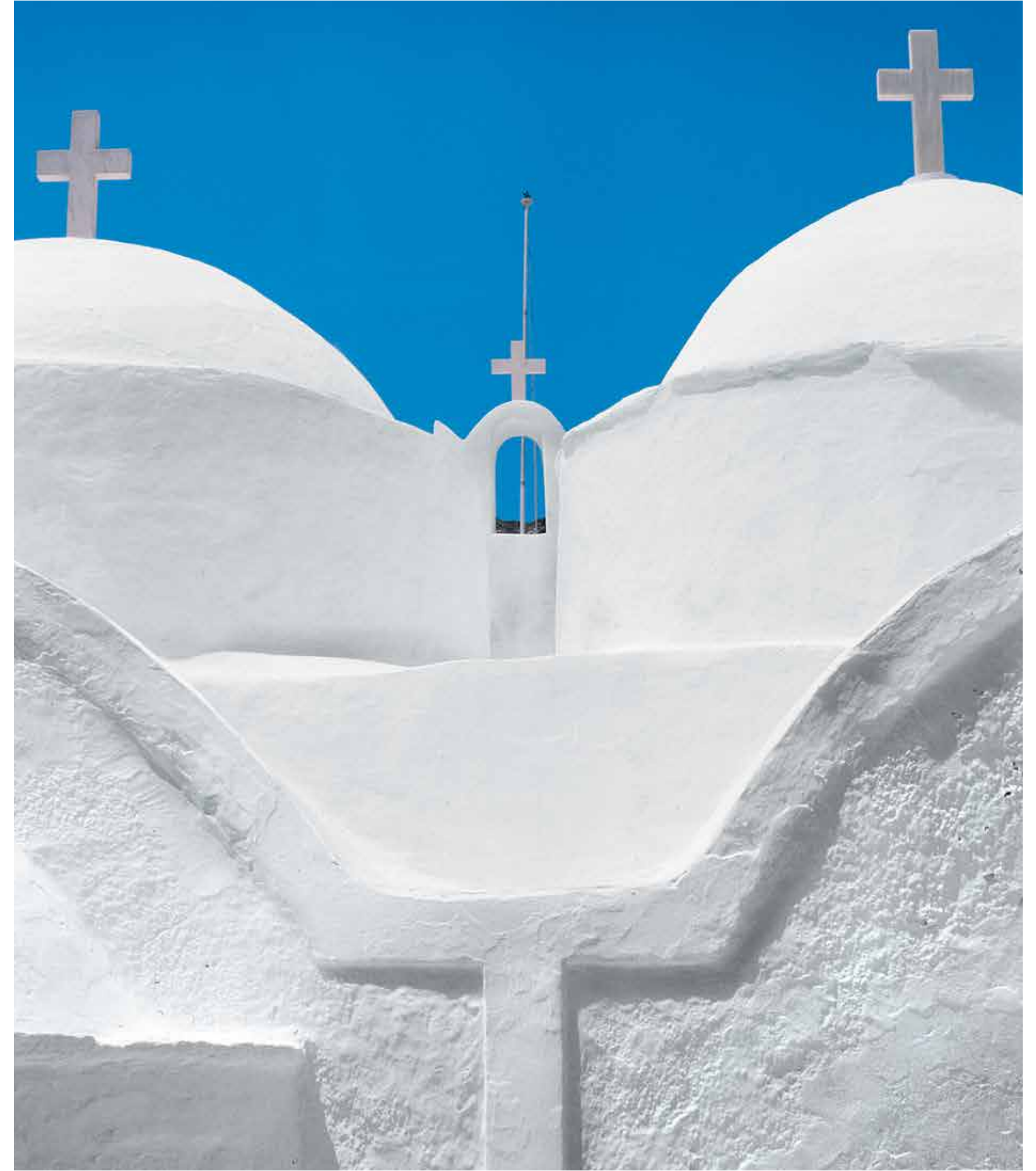
Two single-nave-with-dome chapels joined into one in Vathi, Sifnos. The view is to the west, and the cross in the middle sits on top of the shared bell tower, an upward extension of the west entry wall to the chapel.
