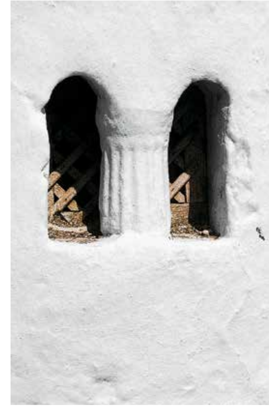
Astypalaia. A double-apse window of moderate size allows limited light to enter, adding some gentle natural illumination to the candlelit interior of the chapel.
