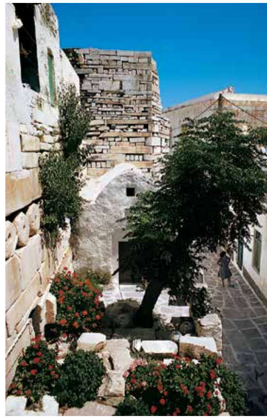
Paroikia. Architectural parts of the nearby ancient Greek temple were reassembled during the thirteenth century to produce the medieval defense tower of Kastro. The houses on the left sit on top of the medieval defense enclosure. The church of Ayia Anna and its small front patio incorporate architectural fragments. The medieval tower in the background, as well as the pedestrian path on the right, also speaks eloquently of the integration of Paroikia Kastro parts into the urban fabric of the contemporary Paroikia town.
