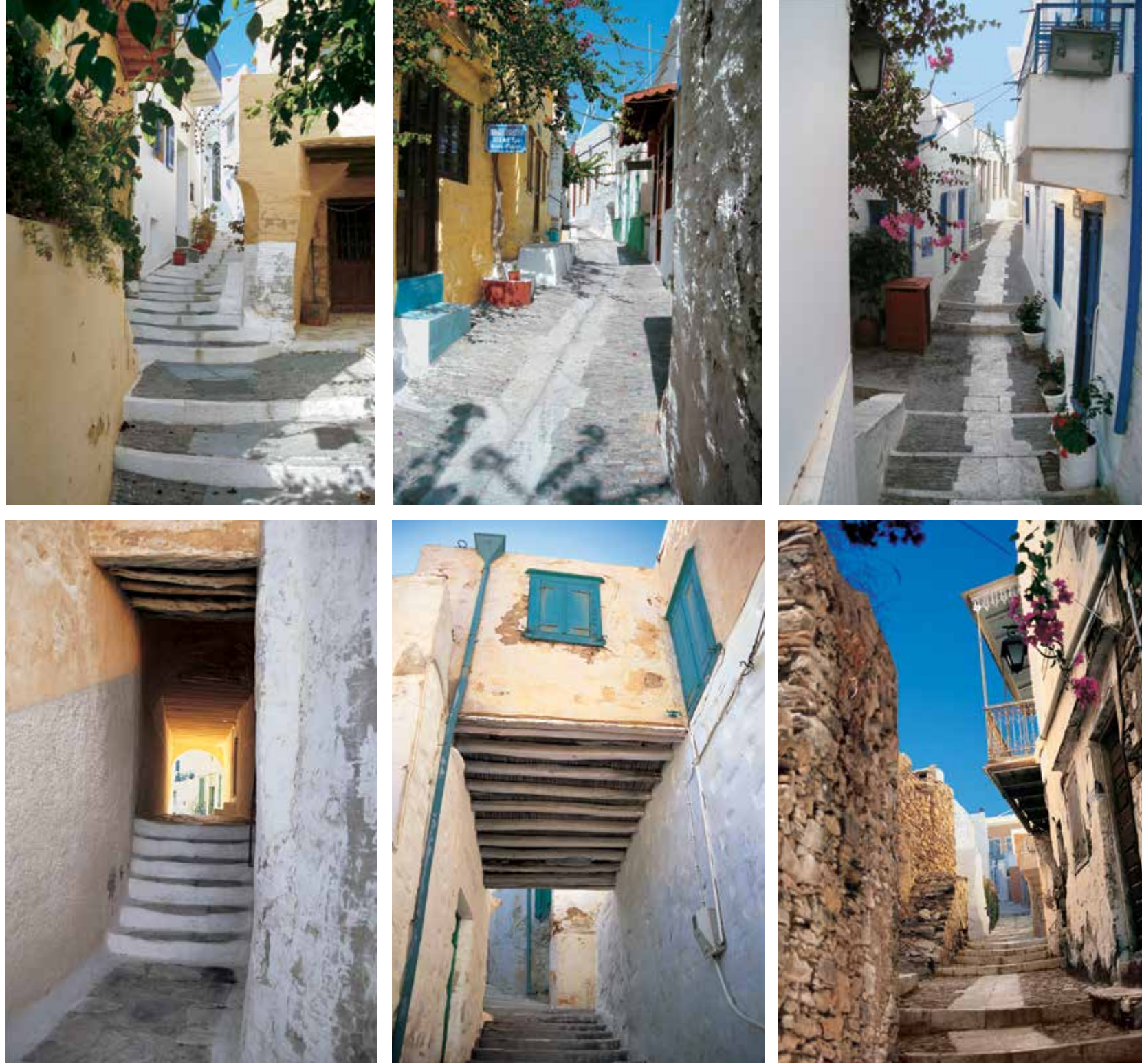
Ano Syros. Pedestrian paths. Typical Aegean Kastro vernacular architecture features are present, such as a forty-five-degree corner cut to accommodate beast-of-burden traffic (upper left), rainwater collection systems (lower middle), covered passages and others.
