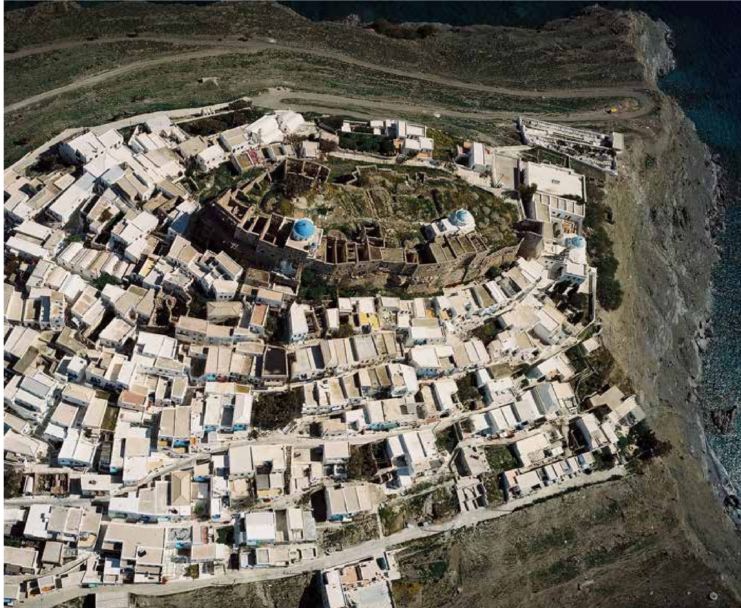
Astypalaia, Kastro and Chora, bird's-eye view. Although they follow the new site's topography and enjoy its amenities, the successive ring-like layers of the dwelling units of Chora nevertheless emulate the typical plan of the older dwelling units inside Kastro.
