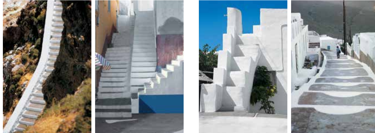
Indispensable elements of the vernacular architecture of the Aegean islands, steps and ramps, mediate ground elevation differences and introduce human scale. The examples are from Serifos, Symi, Sifnos, and Astypalaia.
