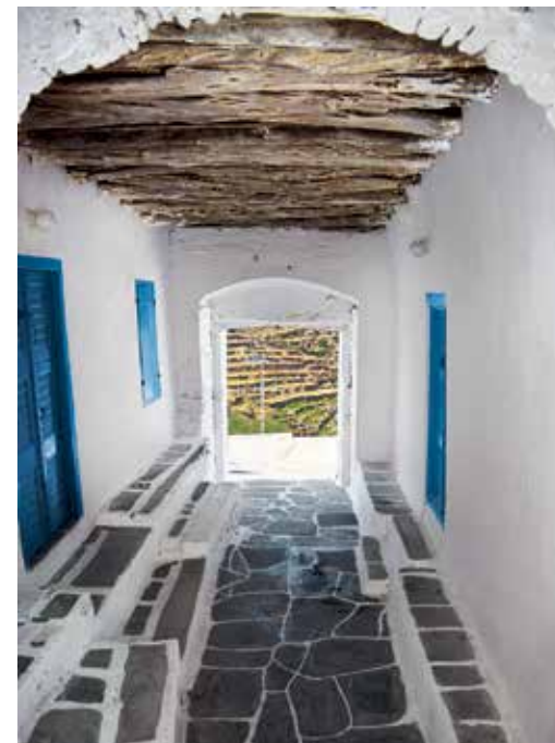
Chandaki gate (inner wall)
