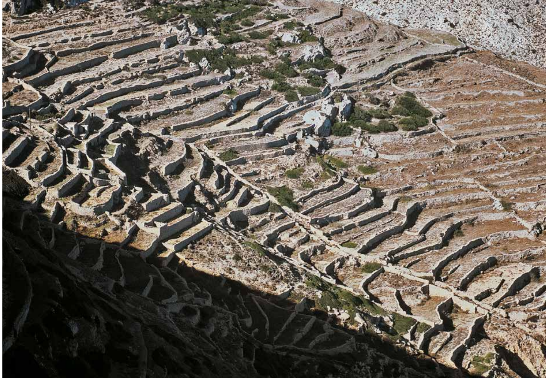
Supporting cultivation and preventing soil erosion for centuries, the retaining walls of Folegandros, above, are inseparable parts of the man-made landscape of the Aegean archipelago and elucidate the observation about the "moderate agricultural wealth" of the islands.
