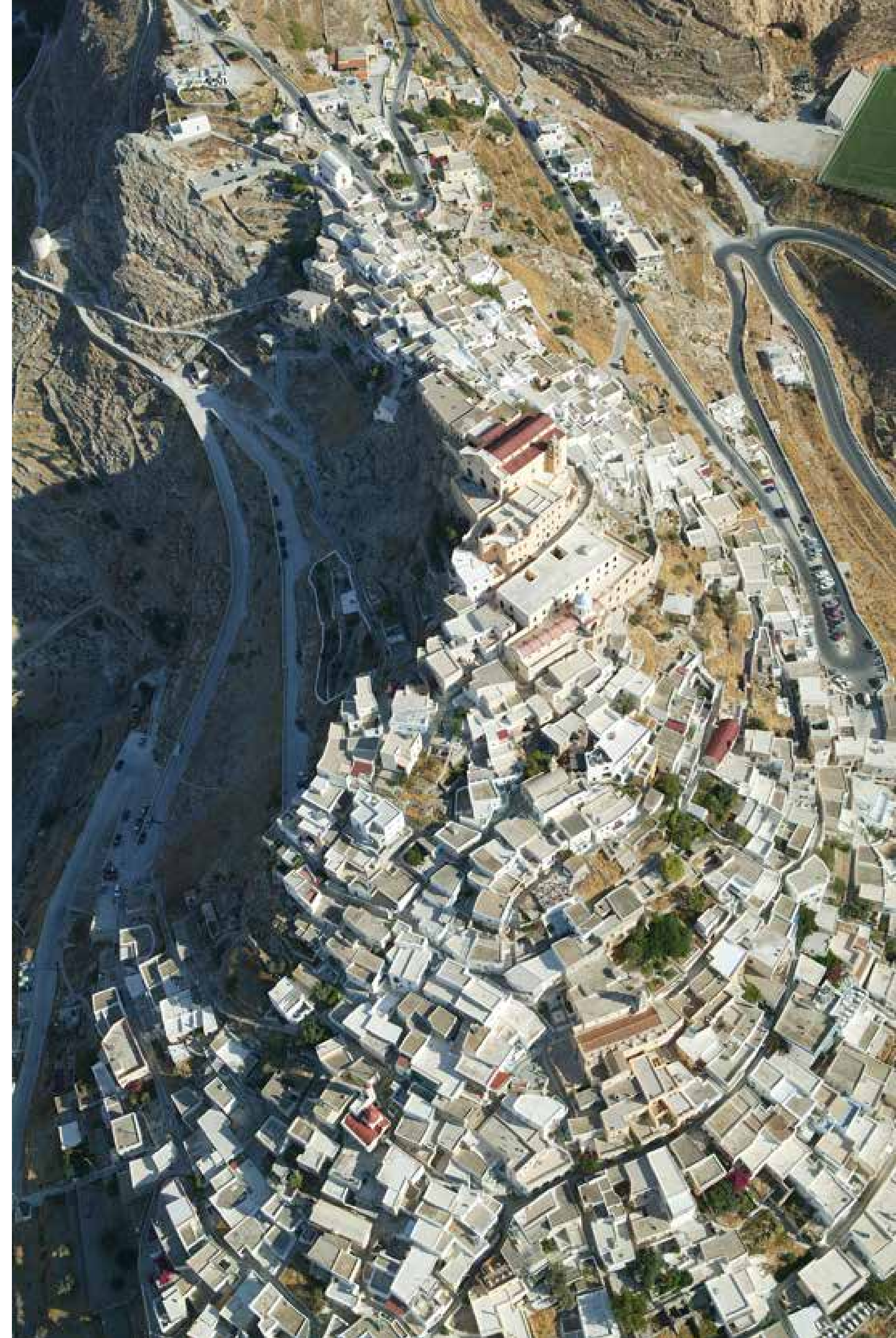
Ano Syros. Helicopter-based photograph revealing the architectural and urban structure of Kastro. The precipitous drop of the northwest half of the site is in shade on the left.
