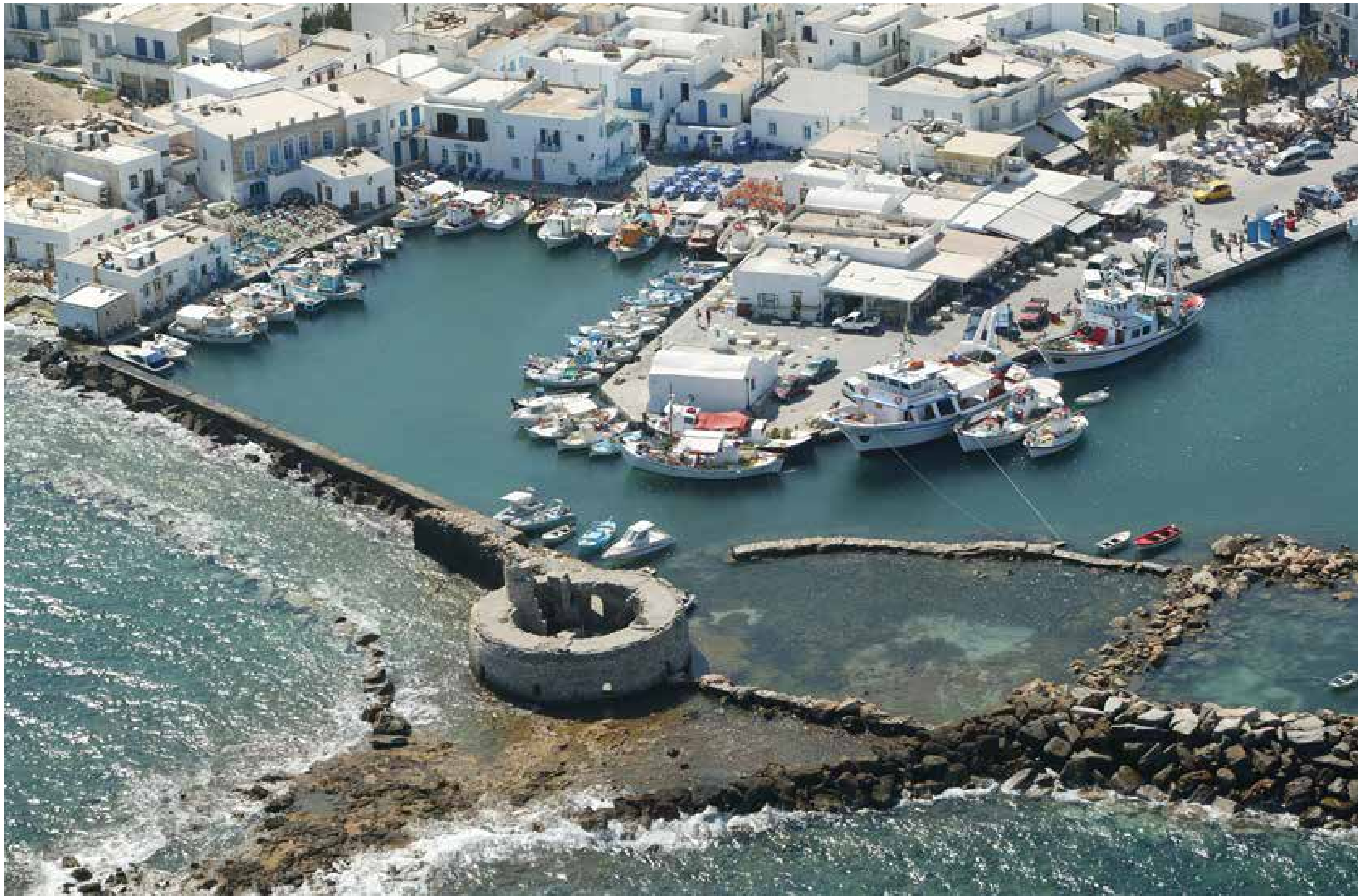
Naoussa, helicopter-based view. The "residential scale" character of the port becomes apparent.
