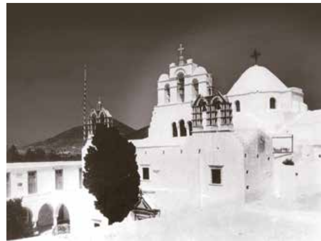
Panayia Katapoliani. This 1948 photograph shows how the Aegean vernacular builders contributed to the architecture of Katapoliani through additions, maintenance and repair work, evident here in the bell towers, whitewash, and the shape of the dome. Restoration work in the 1960s, sought to recapture the glory of the Justinian church of the sixth century A.D. by clearing away vernacular intrusions of the last few centuries.
