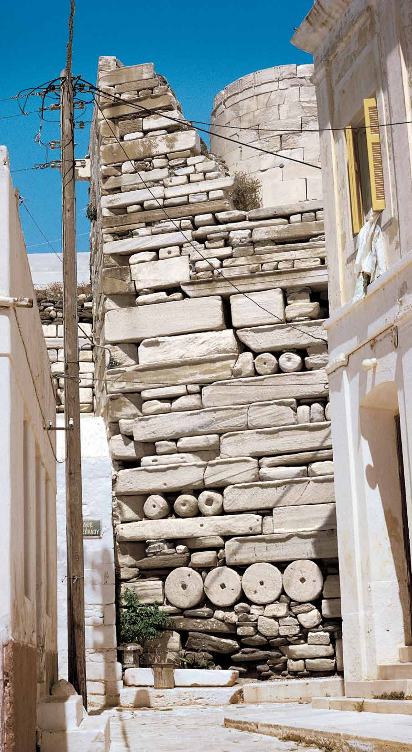
Paroikia. Architectural parts of the nearby ancient Greek temple were reassembled during the thirteenth century to produce the medieval defense tower of Kastro. The houses on the left sit on top of the medieval defense enclosure. The church of Ayia Anna and its small front patio incorporate architectural fragments. The medieval tower in the background, as well as the pedestrian path on the right, also speaks eloquently of the integration of Paroikia Kastro parts into the urban fabric of the contemporary Paroikia town.
