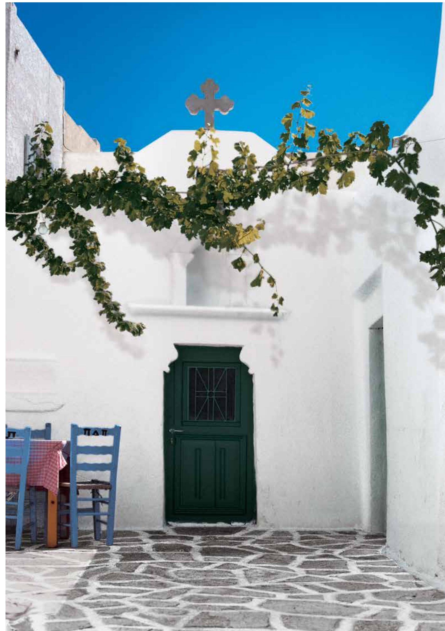
Church incorporated in the later additions to the Antiparos Kastro
