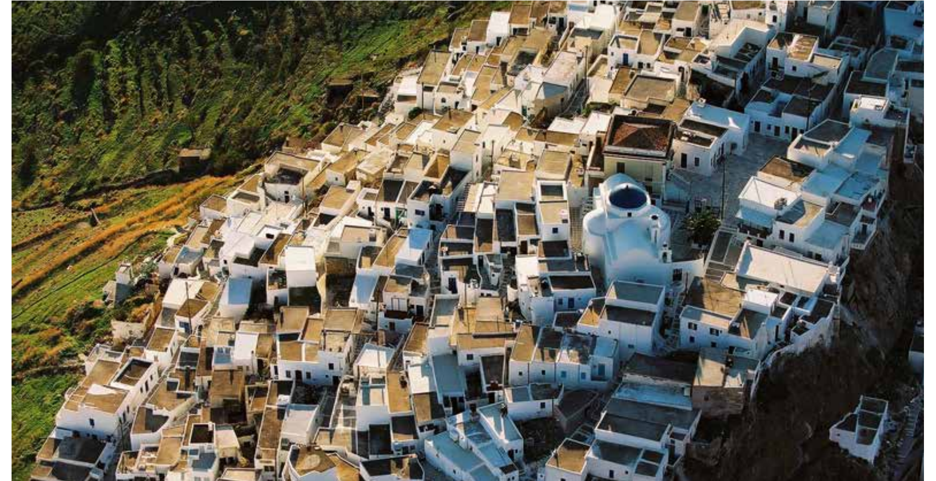
This helicopter-based photograph is of Serifos Chora, built on a visually commanding, two-hundred-meter-high hill where a medieval Kastro existed; today only a few dispersed parts of it are identifiable. The photograph demonstrates the enduring use of the monochoro type outside the confines of a defense enclosure such as that of Sifnos Kastro. In a dry landscape, flat roofs continue to serve as rainwater catchment areas.
