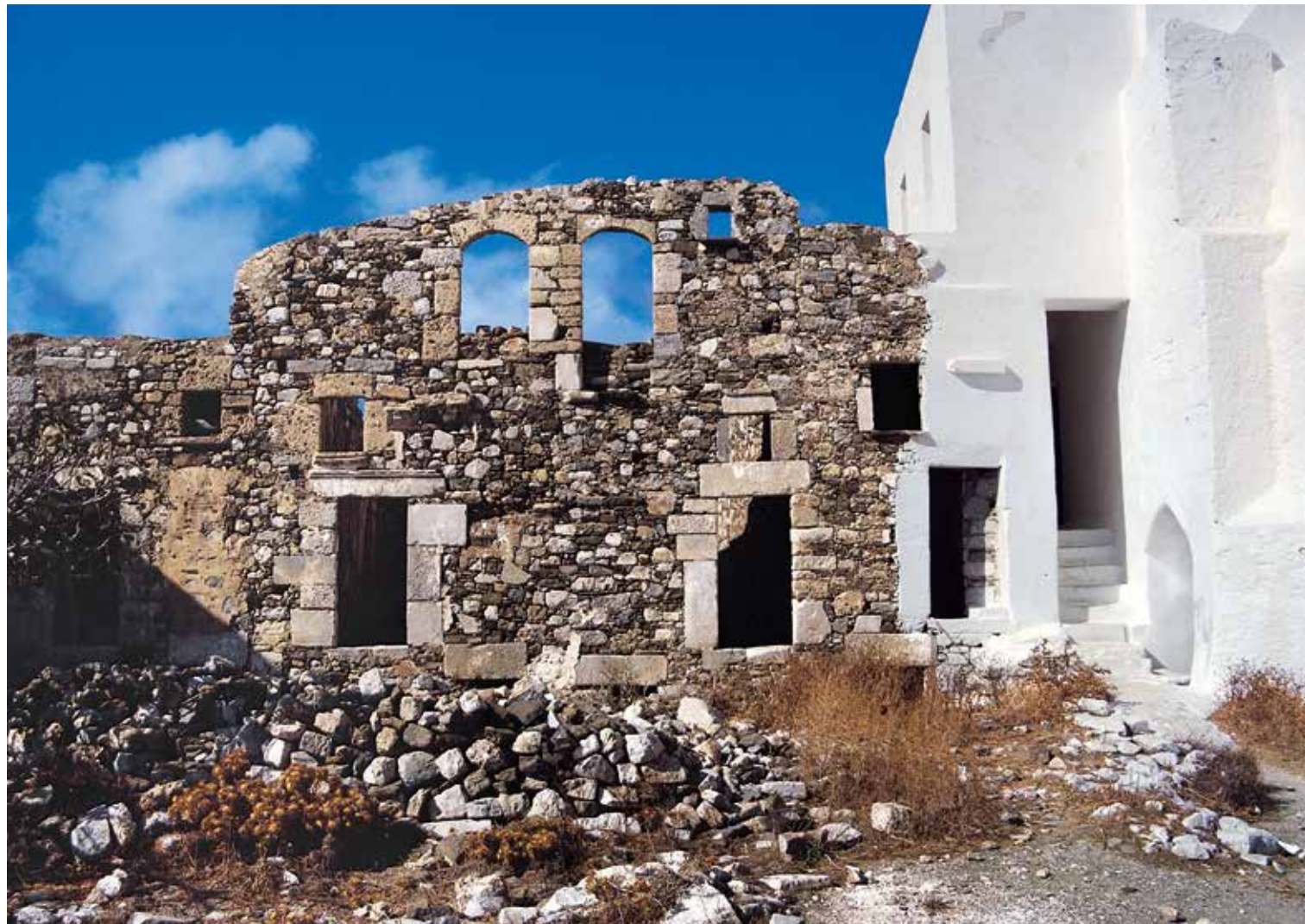
Astypalaia, Kastro, interior walls. The freshly whitewashed surfaces of Panayia church, on the right, contrast with the exposed masonry walls and monolithic lintels of a deserted dwelling unit.
