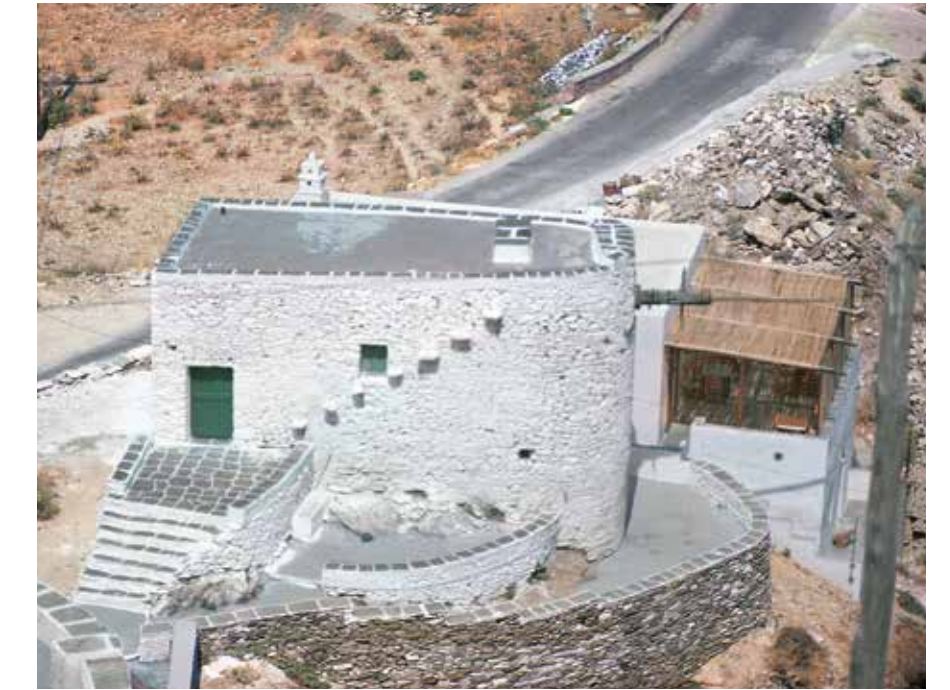
"Horseshoe" type plan windmills using a fixed wind shaft in Olympos, Karpathos (left), and Sifnos, near Kastro (right). The Sifnos windmill has been converted to a house.
