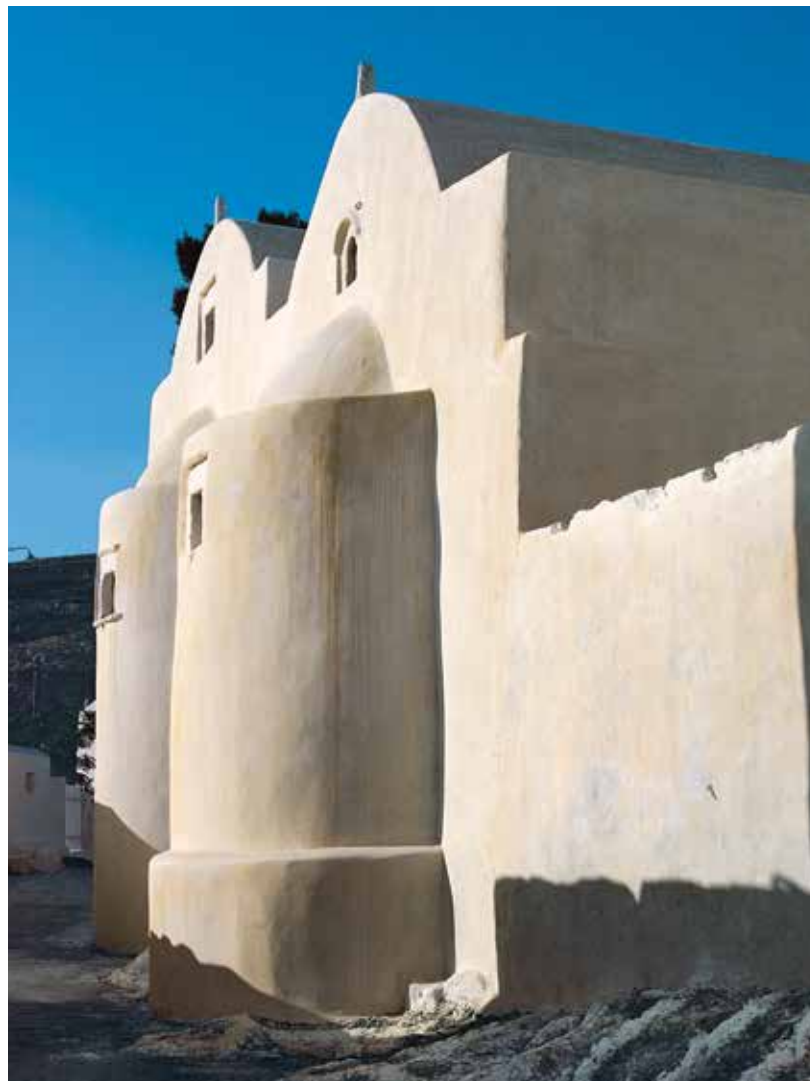
Sikinos Chora. Two single-nave chapels are frequently joined into one building, as the examples on this page illustrate. Some scholars believe that the double-nave, single chapel building originated during the reign of the Duchy of the Archipelago, when the strong Latin Roman Catholic presence in the islands may have prompted a simultaneous double liturgy designed to meet the religious needs of a mixed community. The photograph at the top, looking west during early morning hours, brings to mind Le Corbusier's definition of architecture as "the masterly, correct, and magnificent play of masses brought together in light".
