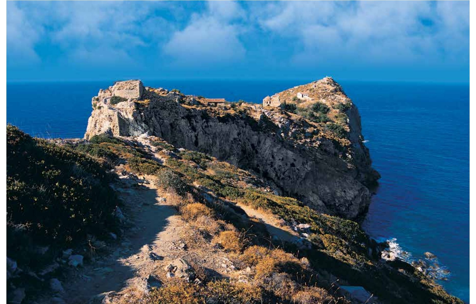
Skiathos, Kastro. Separated by a “deep chasm” from the rest of the island, the gigantic rock at the center of the illustration is the actual site of the medieval Kastro. The site’s surviving buildings, as well as the boundless northern Aegean horizon in the background, attest to the size and scale of this “nest of seagulls.” The drawbridge located on the left corner of the rock is in front of the gate to Skiathos Kastro. The view is to the north and in the direction of Ayion Oros.
