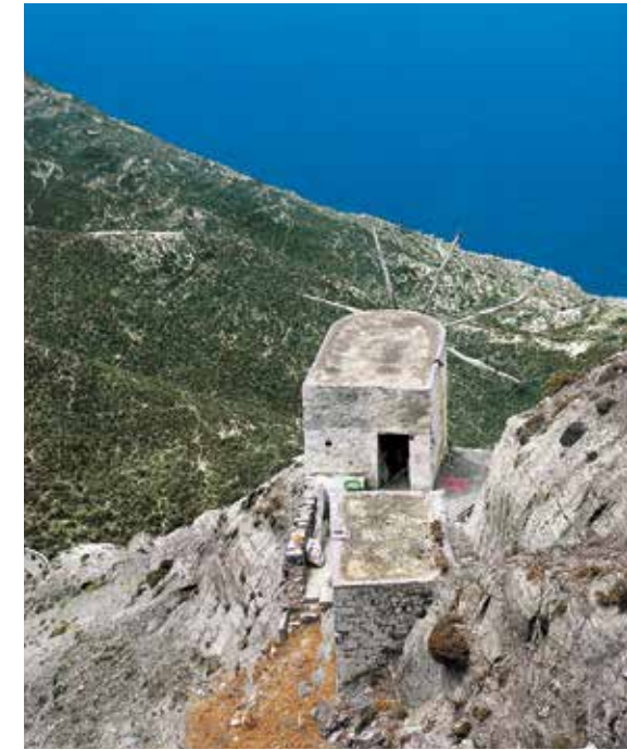
"Horseshoe" type plan windmills using a fixed wind shaft in Olympos, Karpathos (left), and Sifnos, near Kastro (right). The Sifnos windmill has been converted to a house.
