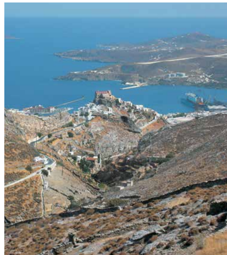
Above: "View of Ano Syros and the Island of Syros." Engraving from "Voyage Pittoresque de la Grece," of Choiseul-Gouffier illustrating economically the mission of the citadel and its relationship to the harbor and landscape of the island. Immediate right: Ano Syros, looking southeast. Note how the hilltop drops precipitously on the side away from the port, thus prohibiting building. The port of Syros appears immediately beyond. Right: Ano Syros. The northwest edge of the hilltop.
