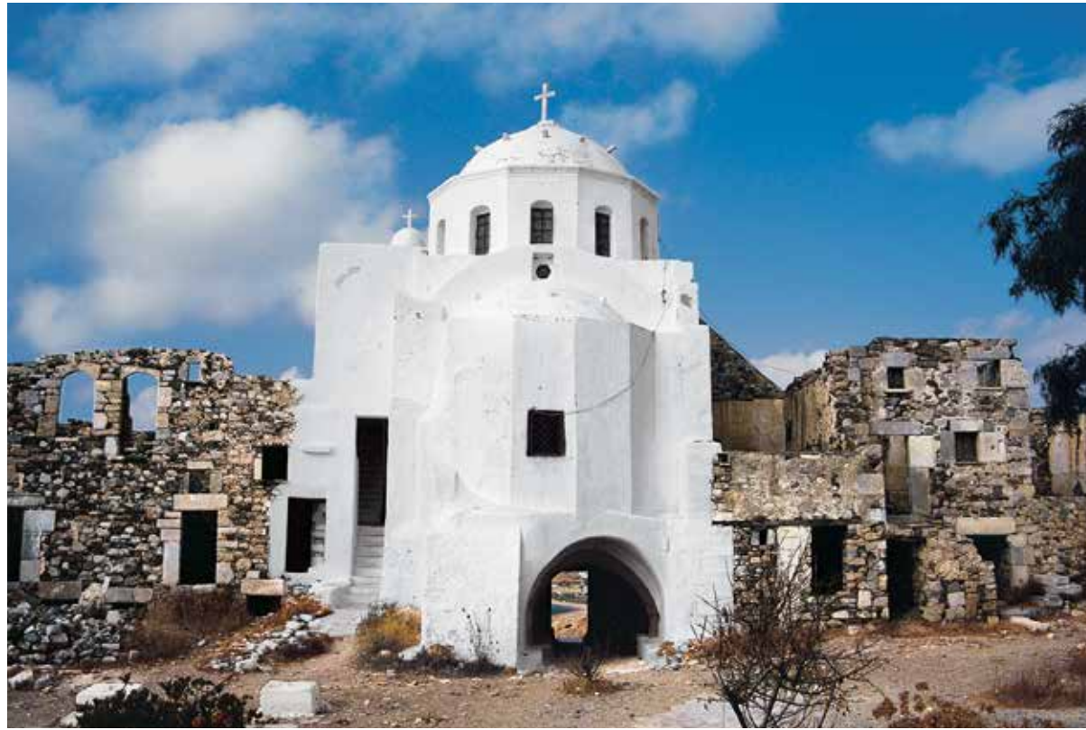
Astypalaia, Kastro. Panayia church sitting above the entry gate, looking west.
