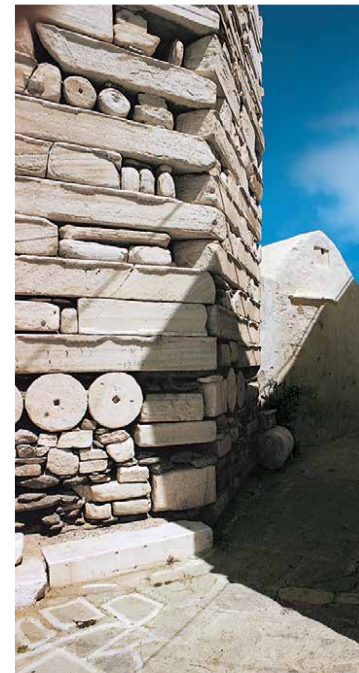
Paroikia. Parts of an ancient Greek temple recycled into the thirteenth century tower.
