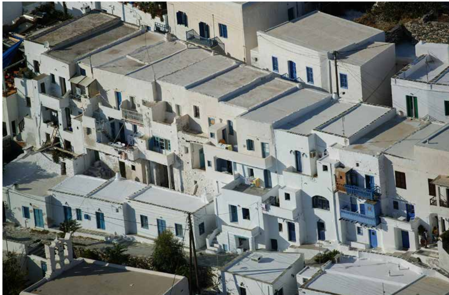
Above: Kastro from the west. The cemetery discussed on page 91 appears at the lower right corner of the illustration. Below: As in other Kastro and throughout the Aegean, the flat roofs of buildings on either side of the Chandaki path have long served as rainwater catchment areas. In this region of limited annual precipitation, drainpipes direct precious rainwater to cisterns often located within the foundation of a house. During the Duchy of the Archipelago days, flat roofs also served, when needed, as continuous ramparts, allowing defenders to move their forces quickly from point to point and to concentrate them as circumstances required.
