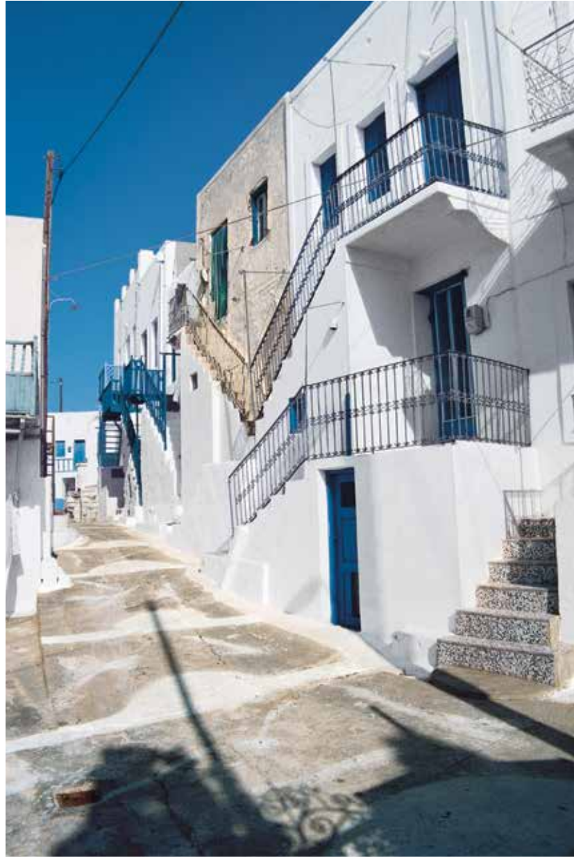
Astypalaia, Chora. Rows of dwelling units flank the spine as it points the way uphill towards Kastro
