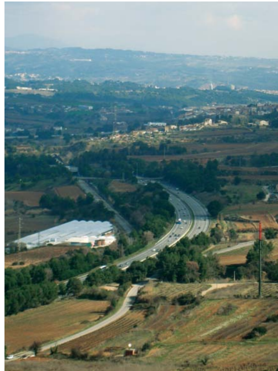
Left: view of the Mediterranean corridor with the motorway AP-7. Right: the system of infrastructures of mobility in the Spatial Plan of the Metropolitan Region of Barcelona.
