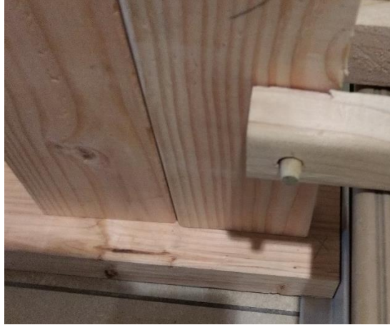
Figure 18 – Dowel Assembly
