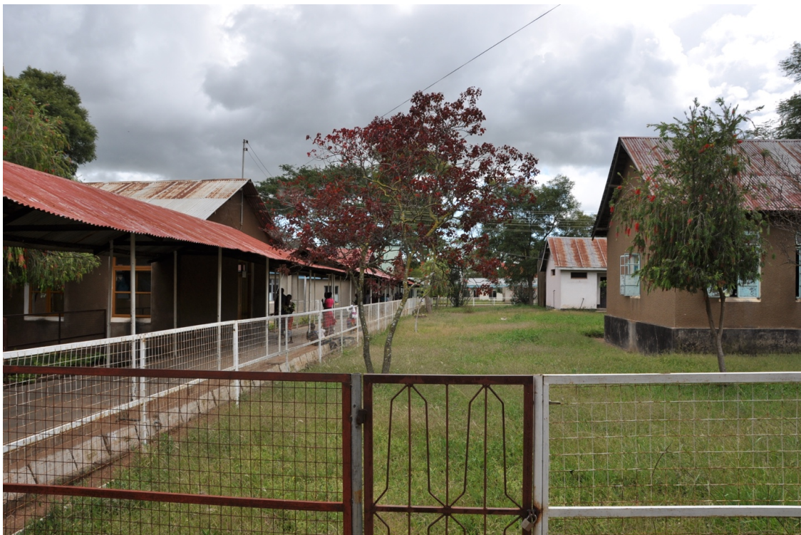
Fig. 5.2 View from inside Mawingu Hospital
