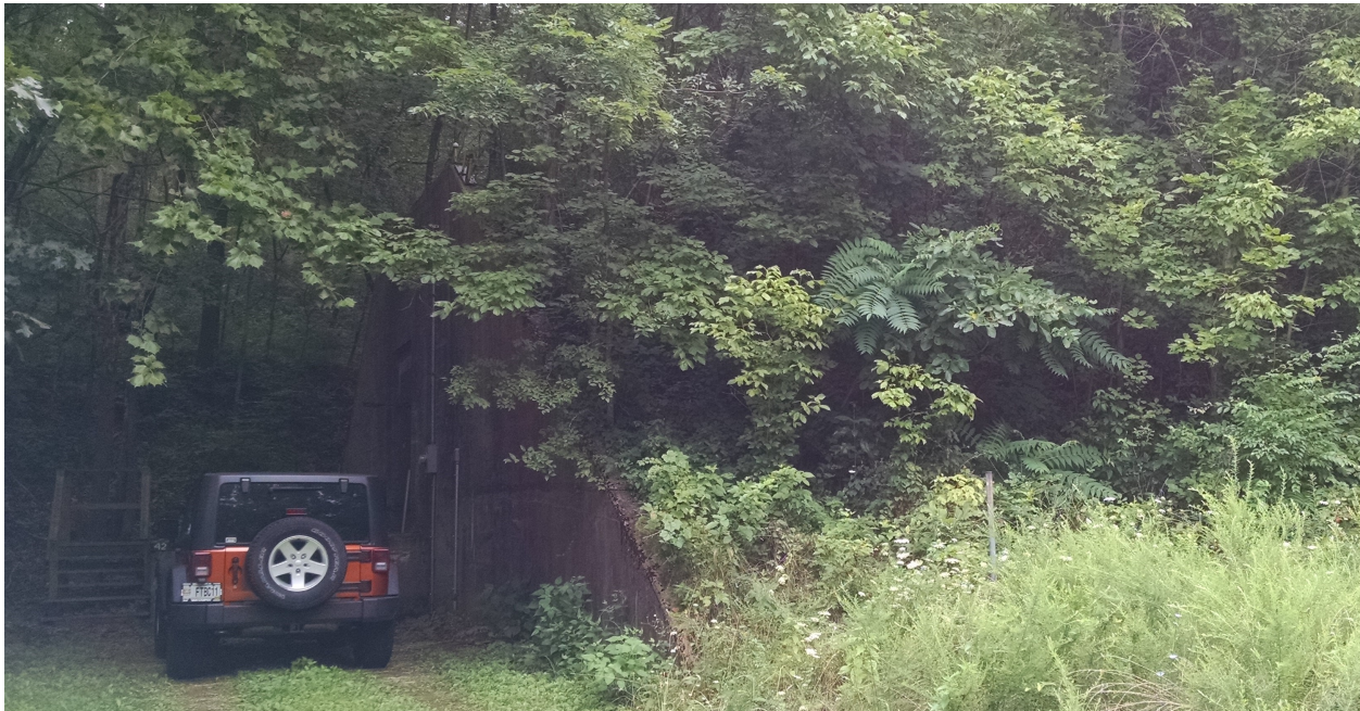
Figure 4.11: Outside view of the bunker. Entrance is just to the right of the Jeep, the bunker extends to the right.
