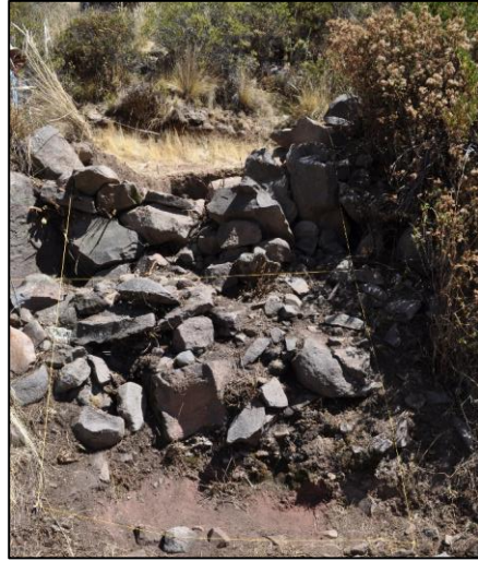
Figure 9.16 : Photo of TZ-3 retaining wall.
