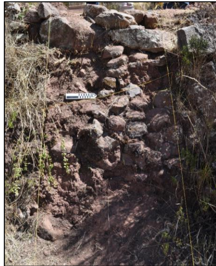
Figure 9.12 : Photo of TZ-6 retaining wall.
