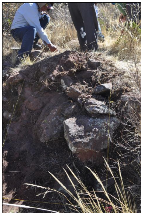
Figure 9.6: Photo of TZ-5 retaining wall.
