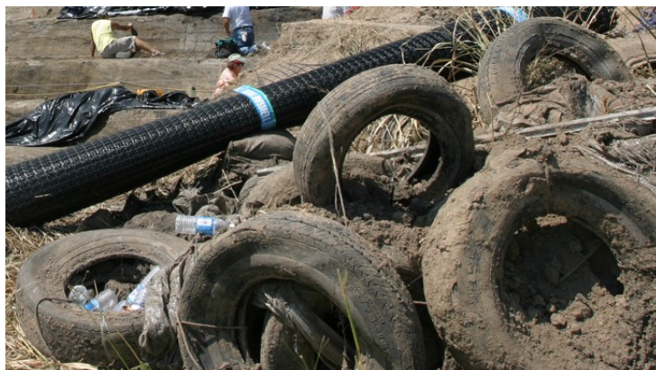
Figure 28. Automotive tires excavated from Face 6.
