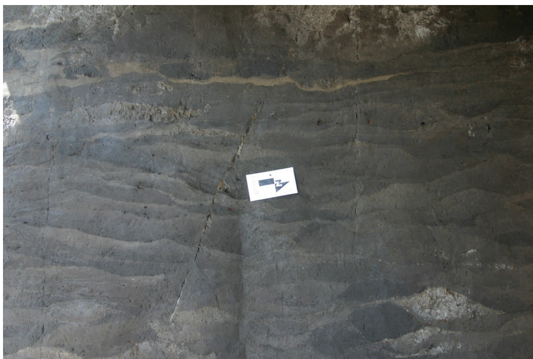
Figure 30. Detail of sod-block construction.
