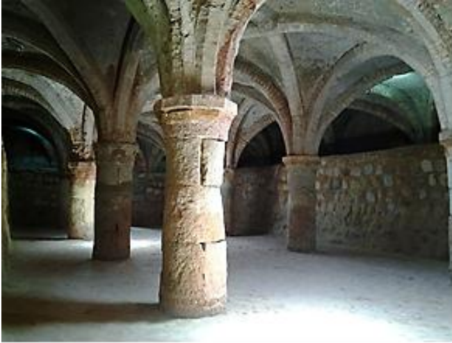
Figure 26. Figure 26. Basement of Portuguese Castle in Hormoz Island (Photographed by: Morteza Golzari).
