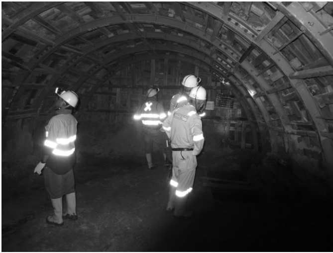
Figure 7. Steel set support installed in GDM underground coal mine roadway.
