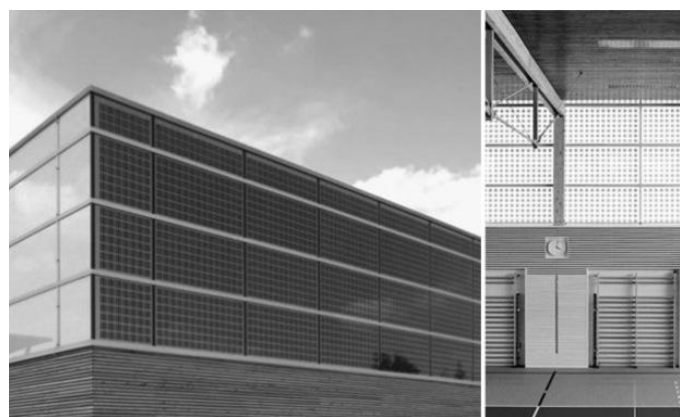
Figure 2. Sports Hall in Burgweinting, Regensburg. internal and external view of the PV translucent façade
