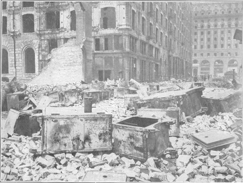
B. ABSOLUTE FAILURE OF SO-CALLED "FIREPROOF" SAFES.
