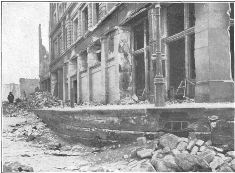
.1. SUBSIDENCE OF STREET IN FRONT OF ÆTNA BUILDING, SAN FRANCISCO.
