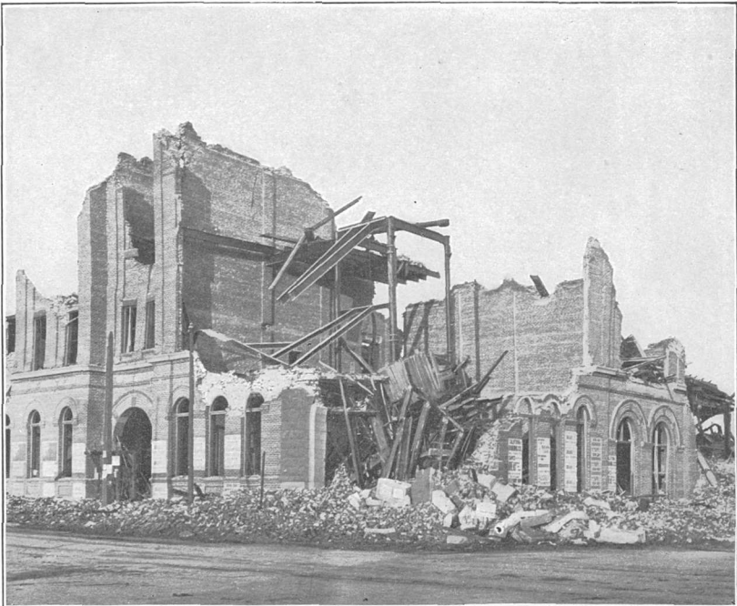
B. EARTHQUAKE DAMAGE, JACKSON BREWING COMPANY'S BUILDING, SAN FRANCISCO.
