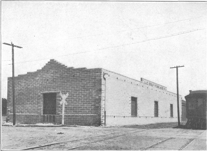
A. ENDURANCE OF WALLS TIED TOGETHER WITH STEEL RODS, LEE BROTHERS' WAREHOUSE, SANTA ROSA.
