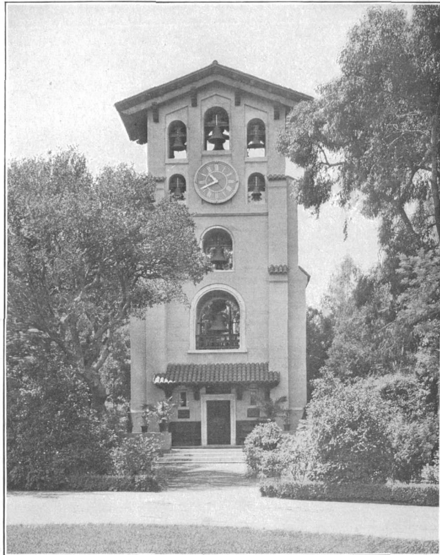
B. UNDAMAGED REINFORCED-CONCRETE STRUCTURE AT MILLS COLLEGE, NEAR OAKLAND.
