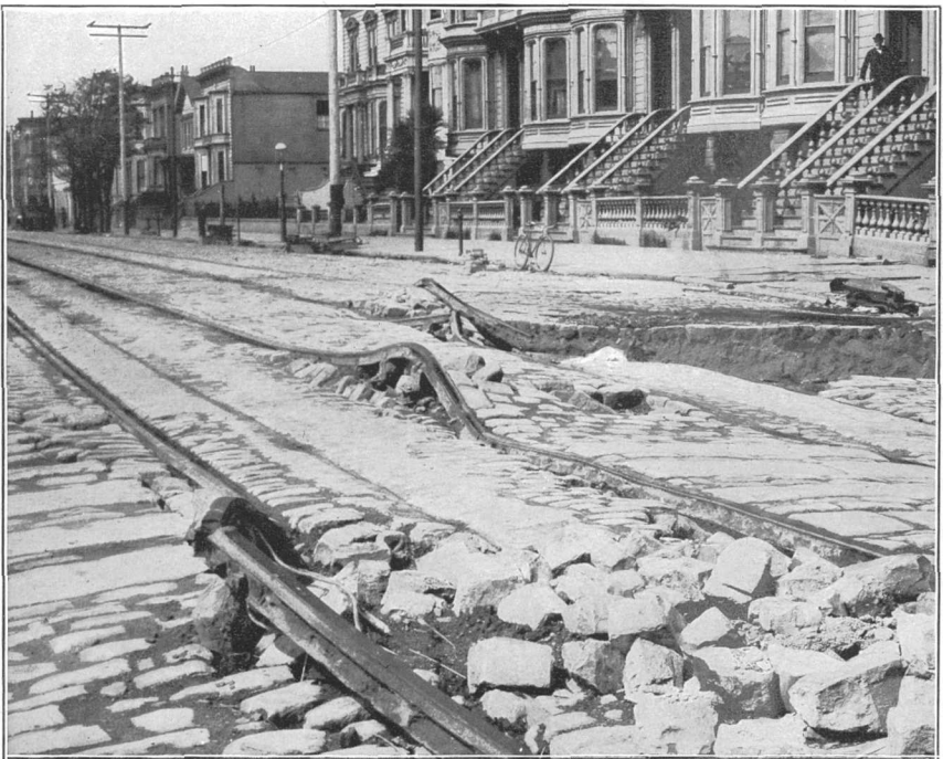
B. BUCKLING CAUSED BY EARTH FLOW, HOWARD STREET, SAN FRANCISCO.
