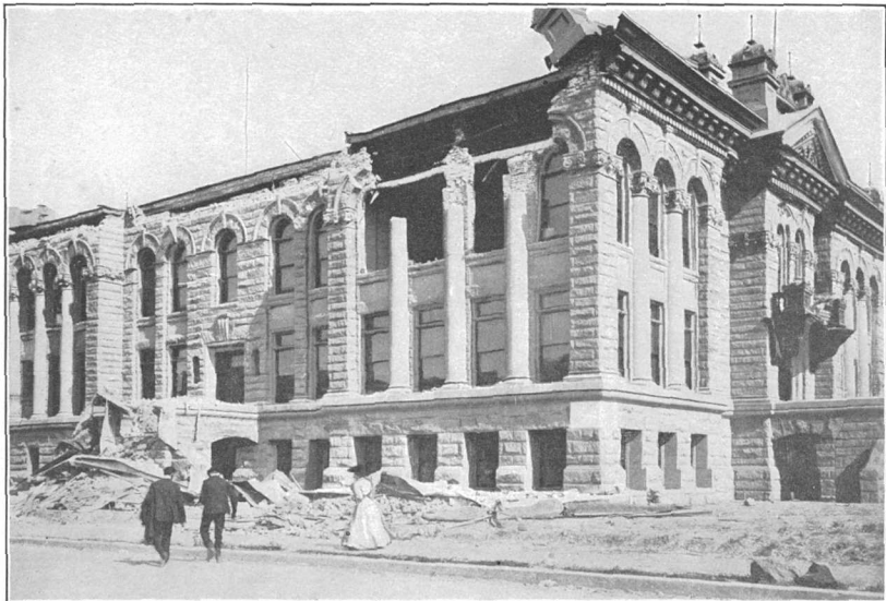
B. EARTHQUAKE WRECK OF NEW HALL OF JUSTICE, SAN JOSE, BUILT ON ALLUVIAL SOIL.
