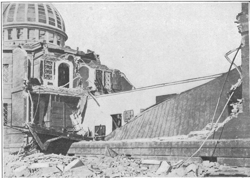
A. COMPARATIVE BEHAVIOR OF REINFORCED CONCRETE AND BRICKWORK UNDER EARTHQUAKE VIBRATION, MUSEUM, LELAND STANFORD JUNIOR UNIVERSITY.
