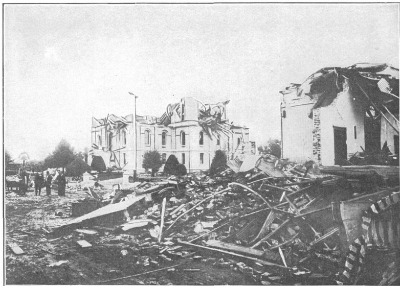
B. COMPLETE WRECK BY EARTHQUAKE, COURT-HOUSE AND HALL OF RECORDS, SANTA ROSA.
