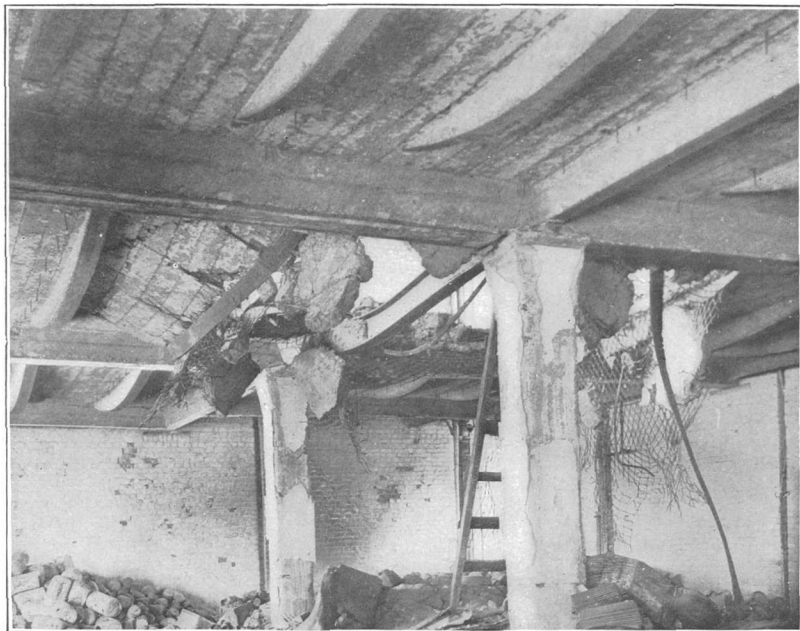
B. COLLAPSE OF FLOOR PANEL, CAUSED BY LOAD FALLING FROM A FLOOR ABOVE, THIRD FLOOR OF ÆTNA BUILDING, SAN FRANCISCO.
